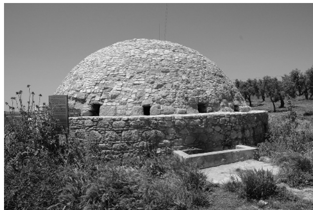
Figure 1.1.8 Ottoman cistern built for military purposes of the Ottoman Army, located near Bodrum, Turkey. (Photos by L.W. Mays)
