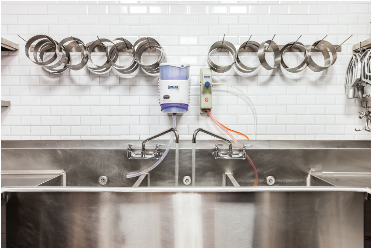
Three-bay sink used to soak, wash, and sanitize small equipment, tools, pots, and tableware.
