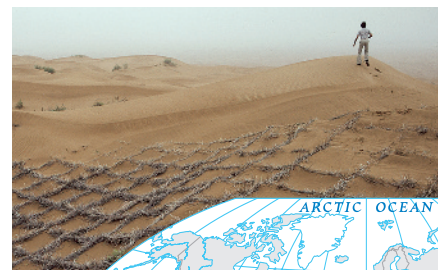
In China's Tengger Desert, sand threatens to engulf nearby railroad lines despite a grid of straw meant to help stabilize the drifts.
