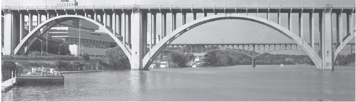
Concrete bridge, Knoxville, Tennessee.
