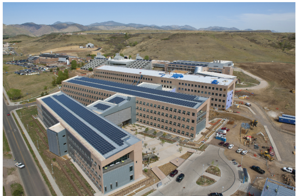
Figure 1.15 The NREL Research Support Facility in Golden, Colorado, is a four-story NZE building that combines low-energy design with high-efficiency photovoltaics to produce all the energy it requires over the course of a year. (Source: National Renewable Energy Laboratory)
