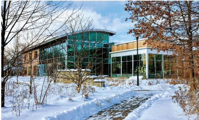
Figure 1.12 The Lewis Center for Environmental Studies at Oberlin College in Oberlin, Ohio, was designed by a team led by William McDonough, a leading green building architect, and including John Todd, developer of the Living Machine. In addition to the superb design of the building’s hydrologic strategy, the extensive PV system makes it an NZE building. (Source: Courtesy of Oberlin College)
