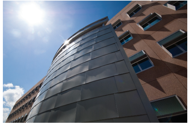
Figure 1.16 Ground view of the air intake structure that conducts outside air into the thermal storage labyrinth in the crawl space of the NREL RSF. (Source: National Renewable Energy Laboratory)
