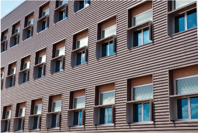
Figure 1.18 The fenestration for the NREL RSF was designed to provide excellent daylighting while controlling glare and unwanted solar thermal gain through the use of shading devices, recessed windows, and electrochromic glass. Operable windows allow the occupants to control their thermal comfort and obtain fresh air. (Source: National Renewable Energy Laboratory)
