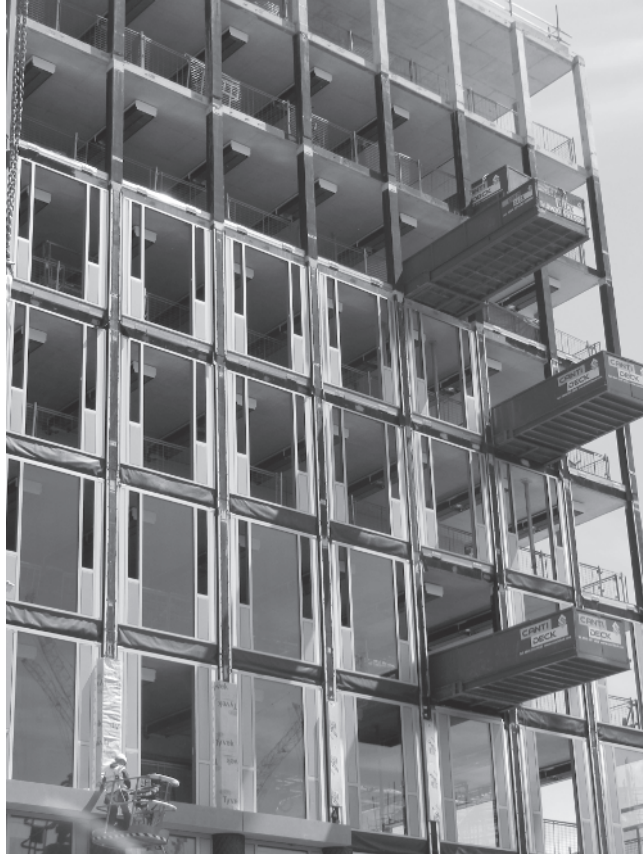
Photograph 1.1 Framed building under construction.
