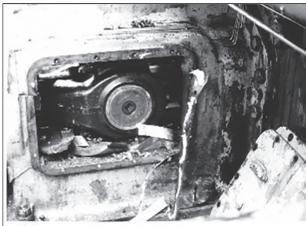
Figure 1.4.1 Wreck of a gas-engine compressor.
