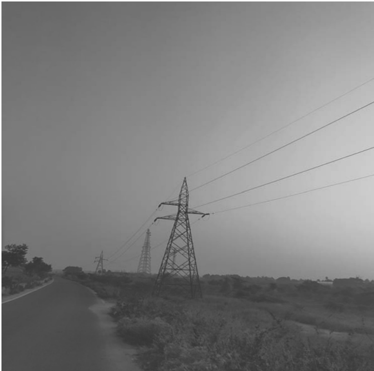
Figure 1.69 Installation of transmission lines 110 kV single circuit.
