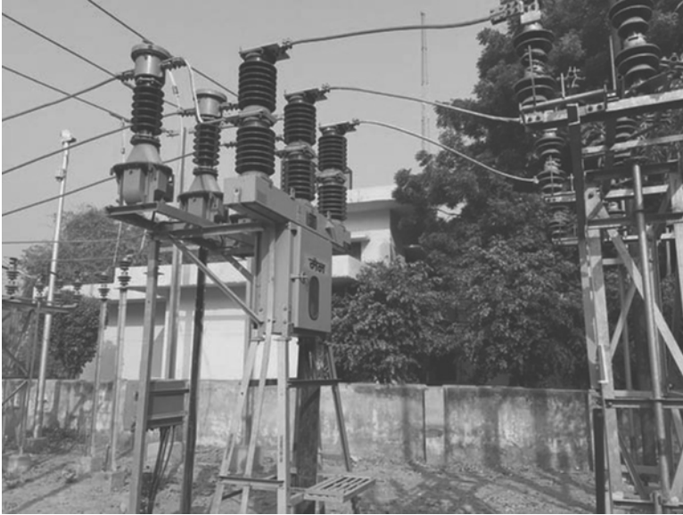
Figure 1.81 Installation of SF 6 breaker.
