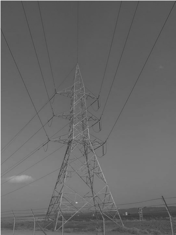
Figure 1.70 Installation of transmission lines 220 kV double circuit.
