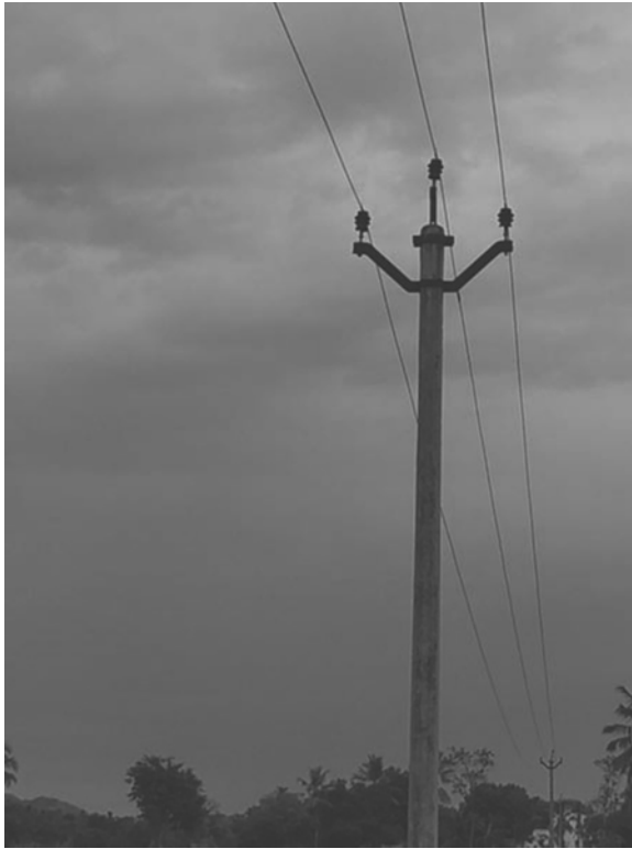
Figure 1.72 Installation of primary distribution line 11 kV single circuit.
