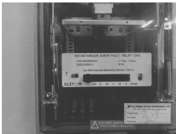
Figure 1.79 Instantaneous earth fault relay (Courtesy: Alstom).
