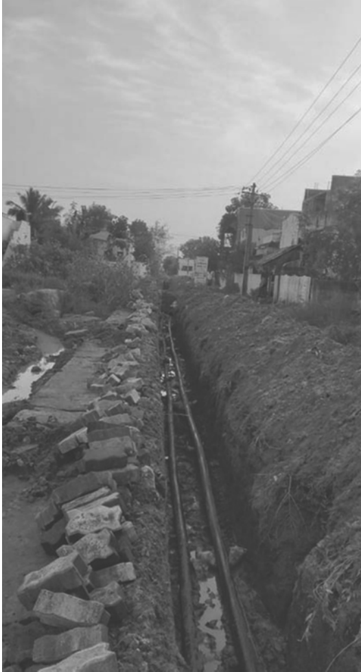
Figure 1.74 Installation of underground cables in buried cable trench.
