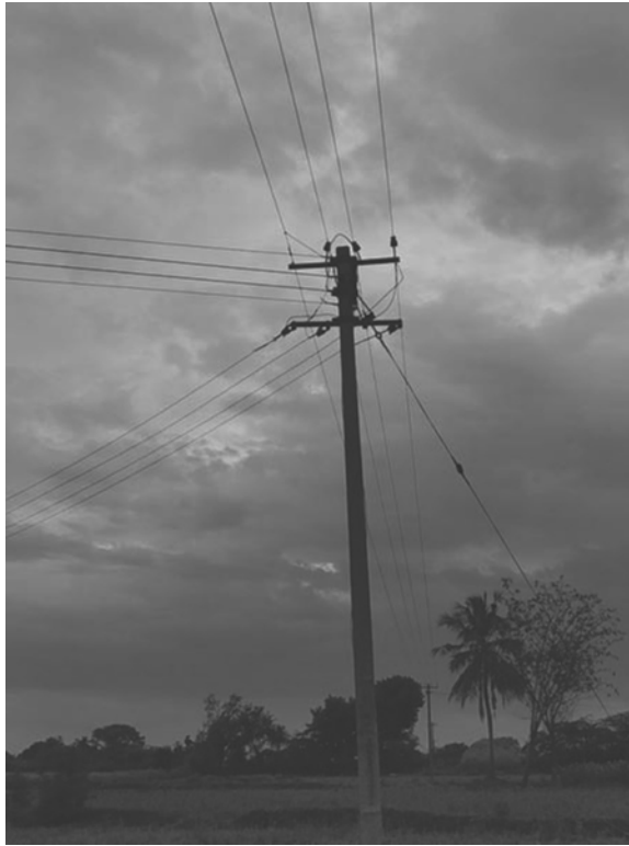
Figure 1.73 Installation of secondary distribution line 415 V.
