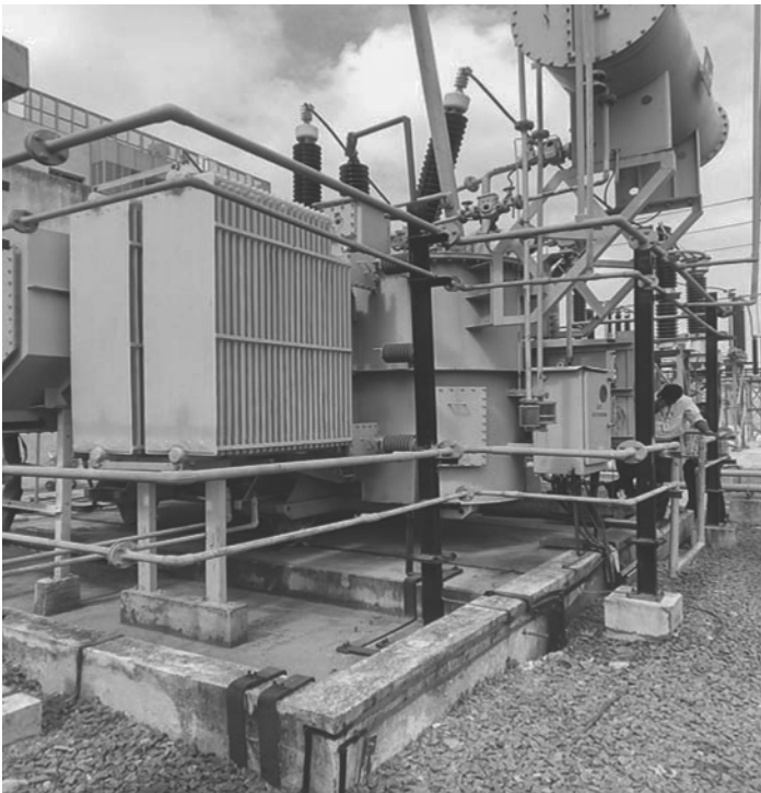
Figure 1.68 Installation of transformer at actual site.
