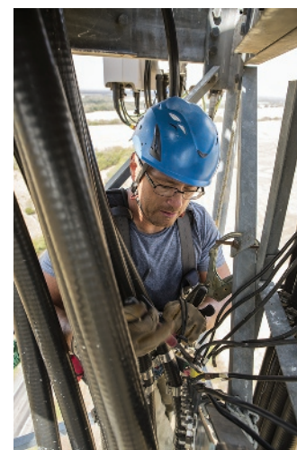
Shannon Faulk/DreamPictures/Getty Images A poor connection in a transmission cable can cause a discontinuity in the electrical signal it carries.
