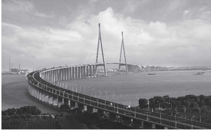
Figure 1-7 Sutong Bridge in Suzhou, Jiangsu, China (Photo provided by Xiaoyan Liu)
