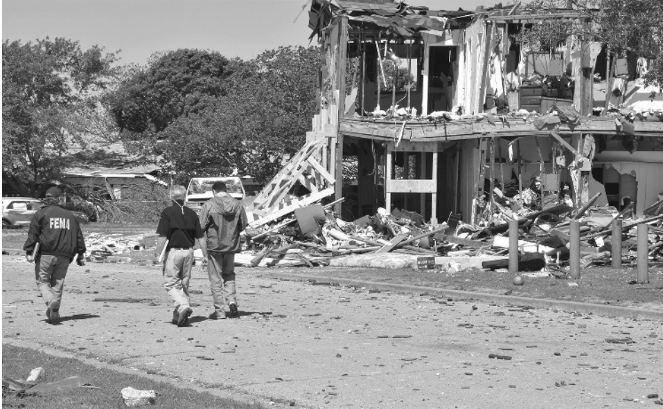
Figure 1-6 The April 20, 2013, West Texas fertilizer plant explosion produced major damages, including to this apartment complex. Earl Armstrong/FEMA. http://www.fema.gov/media-library/assets/images/70270
