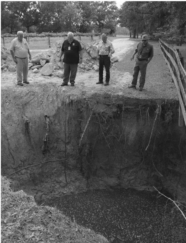
Figure 1-4 This 45-foot deep sinkhole formed in Monticello, FL, after Tropical Storm Debby produced excessive rains and flooding. David Fine/FEMA.
