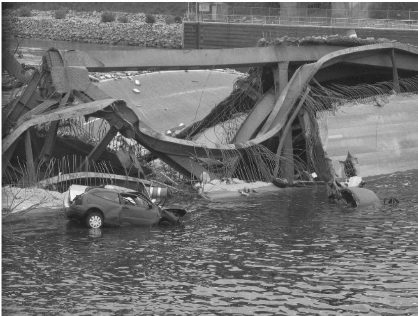
Figure 1-7 The aftermath of the I-35W bridge collapse is seen in this picture from Minneapolis, MN. Todd Swain/FEMA. http://www.fema.gov/media-library/assets/images/51546
