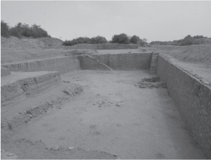
Figure 1.3 Instance of planning in Dholavira. One of 16 water baths surrounding the city perimeter that served as both storage and protection. Courtesy of Uma Edulbehram.
