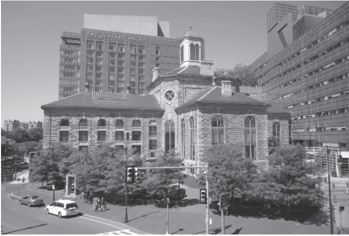
Figure 1.12 Suffolk County Jail in Boston, Massachusetts converted into high-end Liberty Hotel.
