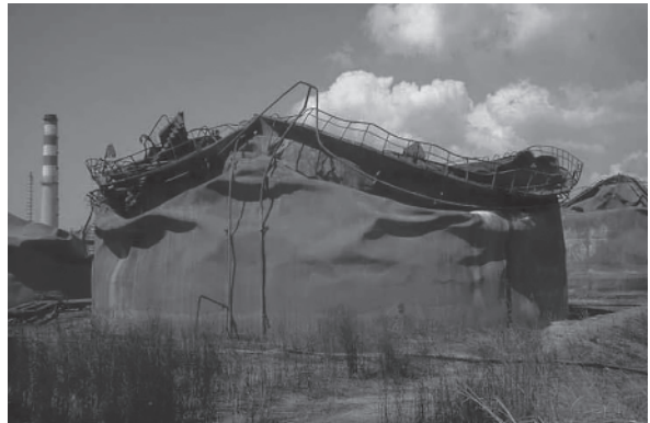
Figure 1.13 Burned tanks following the Izmit earthquake in the Kocaeli Province of Turkey (17 August 1999, Magnitude 7.4). Source: From [573]/Taylor & Francis.
