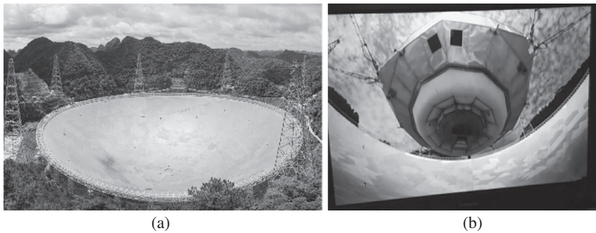
Figure 1.8 FAST 500 m largest radio telescope. (a) Bird's view of the FAST telescope. (b) Feed cabin and cable system.
