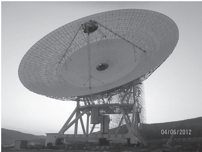
Figure 1.2 A 66 m-S/X-beam guide antenna for Mars detection.
