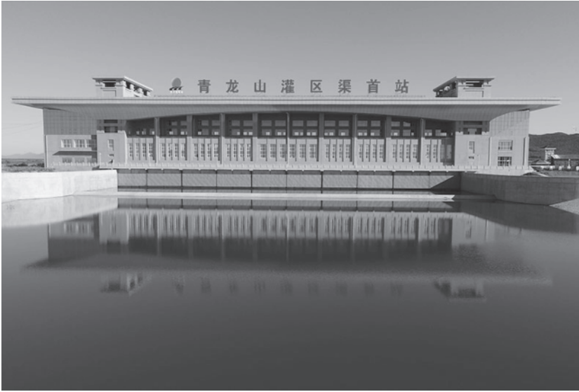
Figure 1.4 Qushou pumping station of Qinglongshan irrigation area in Heilongjiang Sanjiang Plain, China. Source: [3]. Jiangsu Aerospace Hydraulic Equipment Co., Ltd. https://www.pumpcj.com/case/97.html . Last accessed 17 January, 2024.
