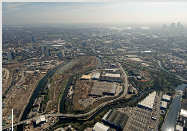
Looking south over the Olympic Stadium 'island site' towards Canary Wharf in April 2007 just as demolition and clearance commenced. The Aquatics Centre on the left of the image was the first to start on site.
