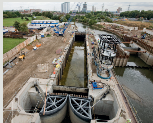
Construction of the new Three Mills Lock on the Prescott Channel in September 2008. It enabled around-the-clock access to the Park for construction barges.
