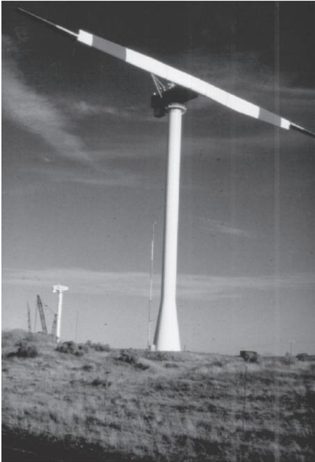
**Figure 1.11** MOD 2 in the Goodnoe Hills (USA): 2.5 MW nominal output, 91 m rotor diameter, 61 m hub height
