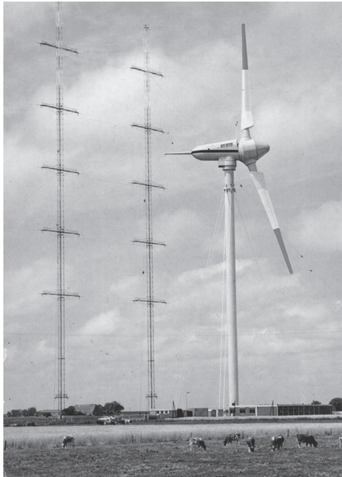
**Figure 1.13** GROWIAN by Brunsbüttel/Dithmarschen, 3 MW capacity, 100 m rotor diameter, 100 m hub height
