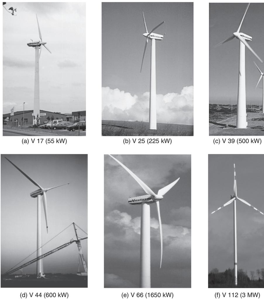
**Figure 1.25** Size progression of Vestas turbines: (a) small, fixed-speed, fixed-pitch machine; (b,c,d) larger variable-pitch units; (d,e) machines with speed elasticity; or double-fed asynchronous generators; (f) machines with permanent excited synchronous generators.
