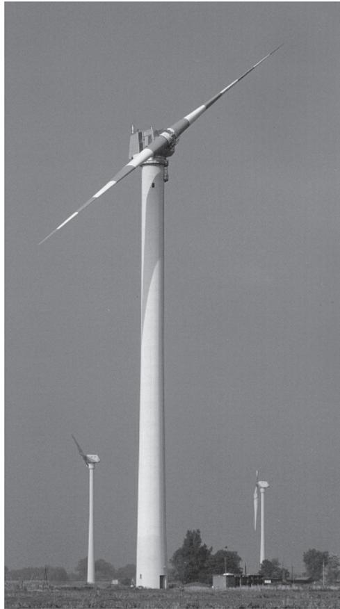
**Figure 1.15** AEOLUS II near Wilhelmshaven: 3 MW nominal output, 80 m rotor diameter, 88 m tower height
