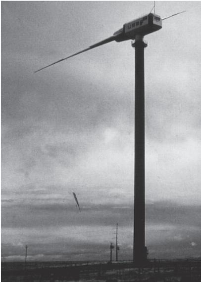
**Figure 1.12** WTS-4 turbine in Medicine Bow, USA.: 4 MW nominal output, 78 m rotor diameter, 80 m tower height
