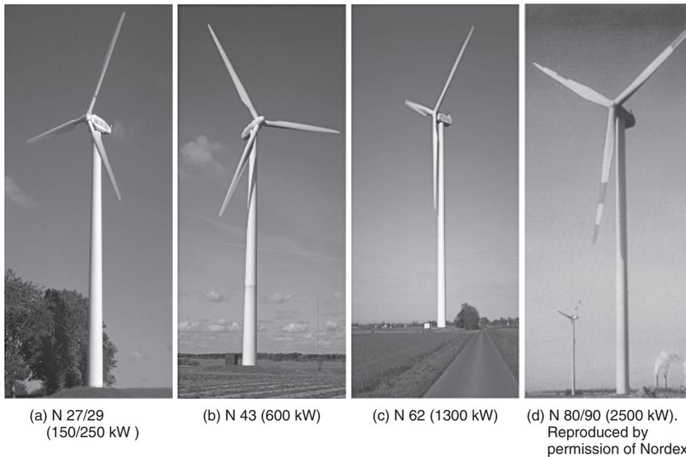
**Figure 1.24** Size progression of Nordex turbines: (a,b,c) fixed-speed, fixed-pitch machines; (d) a large-scale, variable-speed, variable-pitch unit
