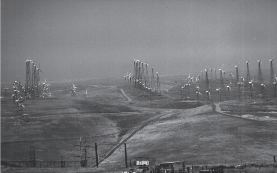
**Figure 1.16** Wind farm in California with turbines in the 50/100 kW class
