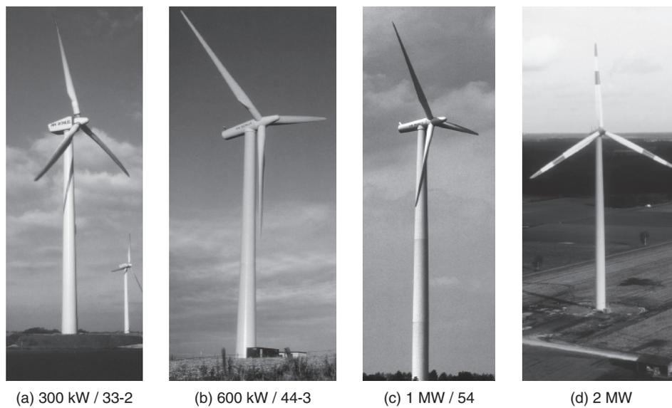
**Figure 1.23** Size progression of Bonus turbines: (a,b) fixed-speed, stall-controlled turbines; (c,d) active (combi-)stall turbines with a slight blade pitch adjustment
