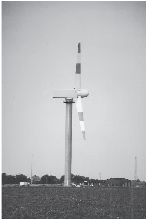
**Figure 1.14** WKA 60 in Kaiser-Wilhelm-Koog: 1.2 MW nominal output, 60 m rotor diameter, 50 m tower height
