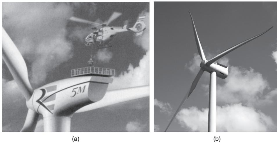
**Figure 1.36** Offshore turbines: (a) Repower offshore and onshore turbine 5M/6M, 5 MW/6 MW nominal output power, 126,5 m rotor diameter. *Source:* Repower; (b) Siemens offshore turbine SWT 6-154, 6 MW nominal output power, 154 m rotor diameter. *Source:* Siemens
