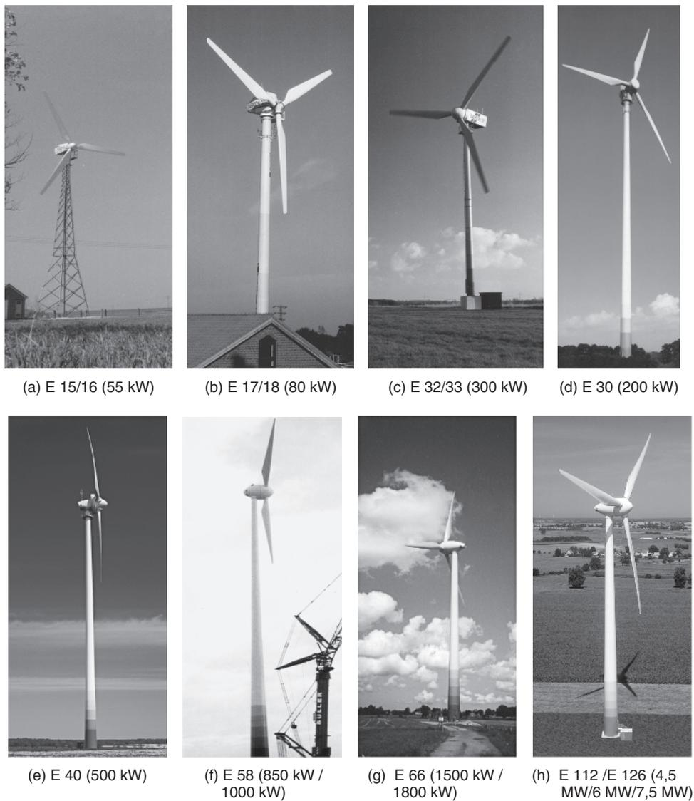
**Figure 1.33** Enercon turbines from variable-speed geared models with thyristor inverters (a,b,c) to gearless configurations with pulse inverters (d,e,f,g,h); (a,b) with fixed and (c,d,e,f,g,h) with variable pitch. Reproduced by kind permission of Enercon
