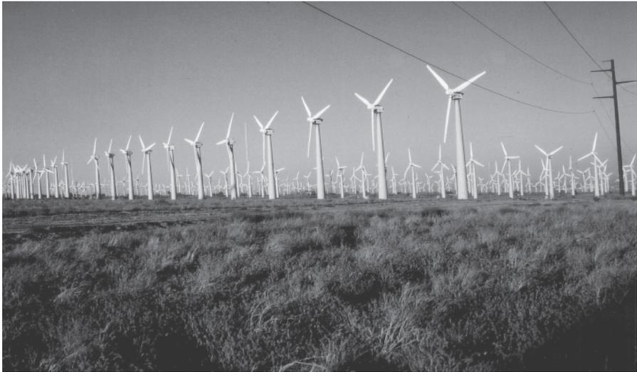
**Figure 1.17** Wind farm in California with turbines in the 250 kW class
