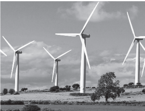
Figure 1.12 A wind farm is a collection of wind turbines connected to the power grid. Each turbine is a complicated engineered system. However, in order to optimize energy production, it is not sufficient to study the individual turbines. Modeling the interactions among the turbines is also important.
