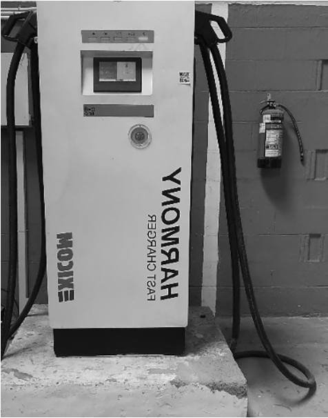
Figure 1.13 DC fast charger 60 kW. Source: Courtesy: EXICOM.
