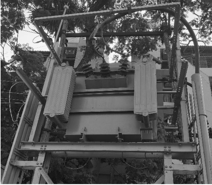
Figure 1.3 Typical distribution transformer.
