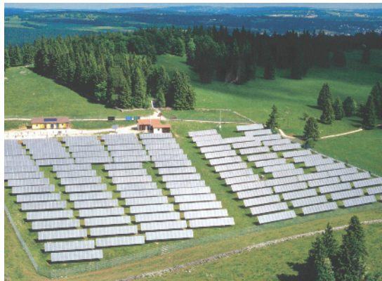
Figure 1.13 The grid-connected 555 kWp system on Mont Soleil, which is located at 1270 m above sea level and was commissioned in 1992
