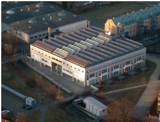
Figure 1.11 A 60 kWp grid-connected system on the roof of the Electrical Engineering Department at Bern University of Applied Sciences in Burgdorf. This installation has been in operation since 1994. © Simon Oberli, www.bergfoto.ch (details from Neville Hankins) (Photo: Simon Oberli)
