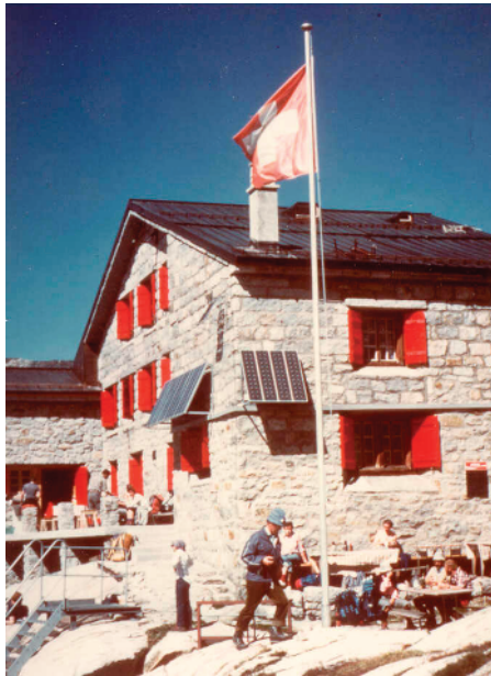
Figure 1.2 The 400 Wp solar generators at the Monte Rosa Hostel in the late 1980s. Such hostels today commonly have PV installations with at least 3 kWp of power (Photo: Fabrimex/Willi Maag)
