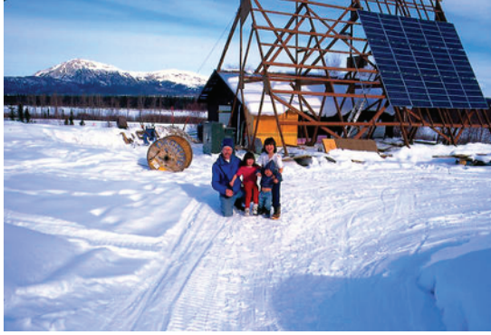
Figure 1.9 PV installation that supplies power to Lime Village, Alaska. This is a 4 kWp stand-alone AC installation with a battery and a backup diesel generator (Courtesy of DOE/NREL)
