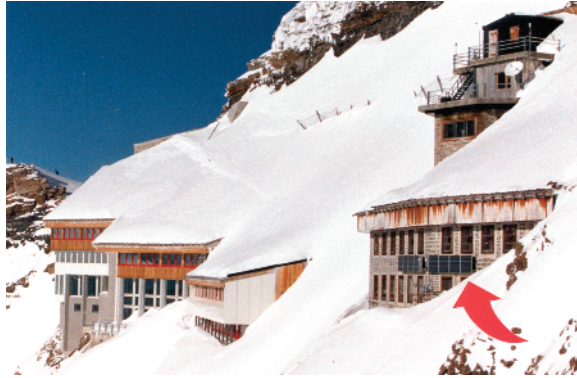
Figure 1.12 The grid-connected system (1152 kWp) owned by Bern University of Applied Sciences on the Jungfrauoch Mountain, which is located at 3454 m above sea level and was connected to the grid in 1993. On inception, the Jungfrauoch facility was the world's highest-altitude PV installation
