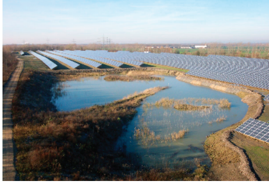
Figure 1.15 The 5 MWp Leipziger Land grid-connected system in Germany that was commissioned in 2004 (Photo: Geosol)
