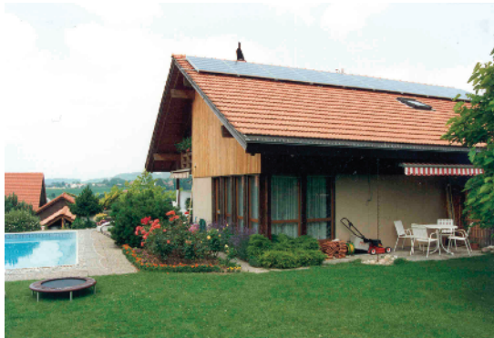
Figure 1.10 A 3.18 kWp grid-connected system on the roof of a home in Burgdorf, Switzerland; the installation has been in operation since 1992
