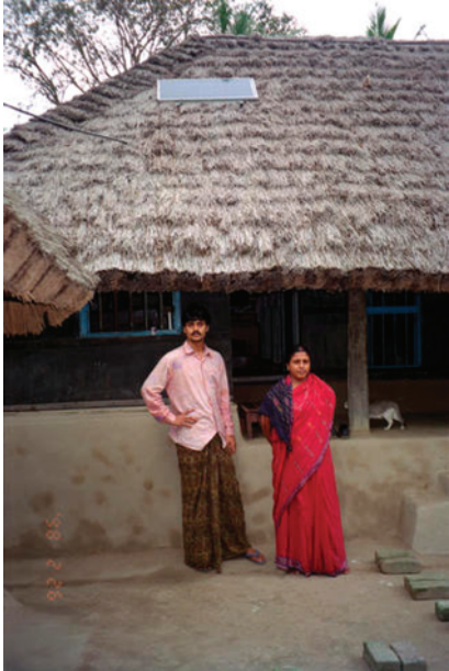
Figure 1.3 Solar home system in India. Even a 50–100 Wp PV installation appreciably raises the standard of living in developing countries (Courtesy of DOE/NREL)
