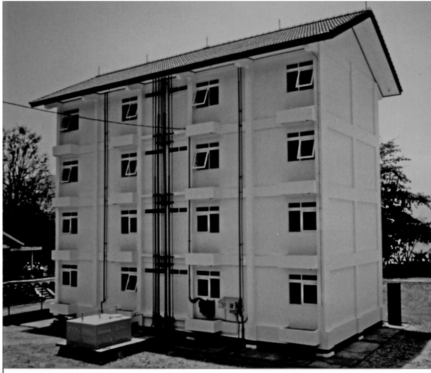
Figure 1.13 Demonstration building in Pelabuhan Ratu, West Java, Indonesia. Courtesy of James M. Kelly. University of California, Berkeley
