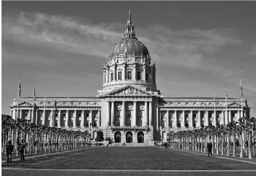
Figure 1.10 The San Francisco City Hall, San Francisco, California. Courtesy of James M. Kelly, University of California, Berkeley
