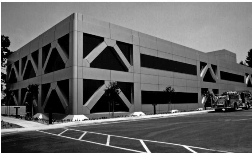
Figure 1.7 Fire Command and Control Facility, Los Angeles, California. Courtesy of James M. Kelly, NISEE Online Archive, University of California, Berkeley
