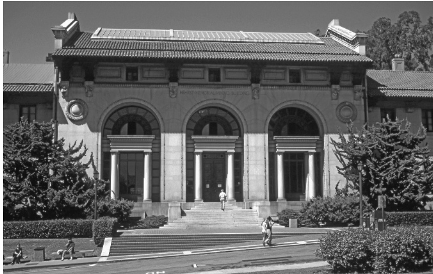
Figure 1.11 Hearst Memorial Mining Building on the University of California, Berkeley campus. Courtesy of Ian D. Aiken, SIE, Inc.
