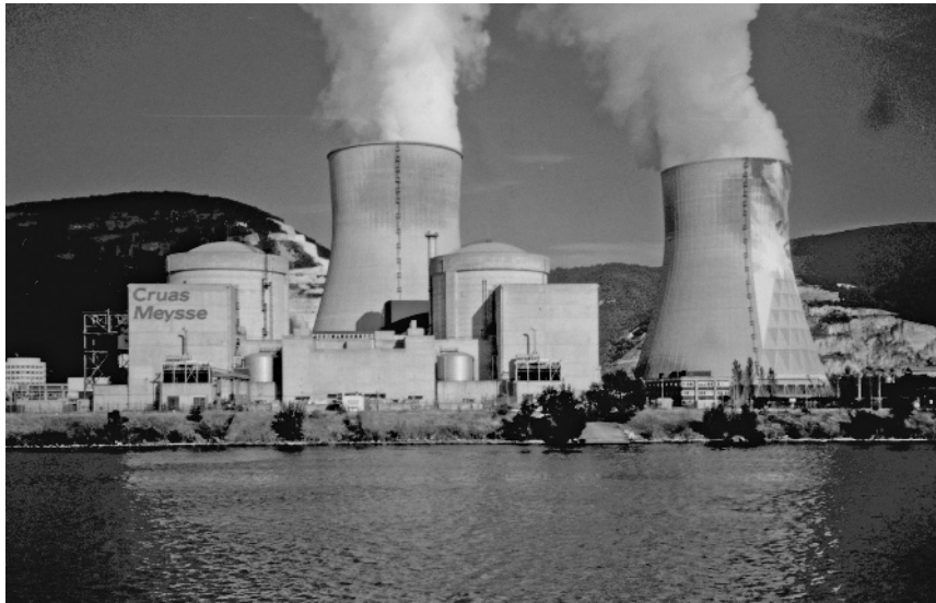
Figure 1.14 The Cruas-Meyssas nuclear power plant. Courtesy of James M. Kelly, University of California, Berkeley
