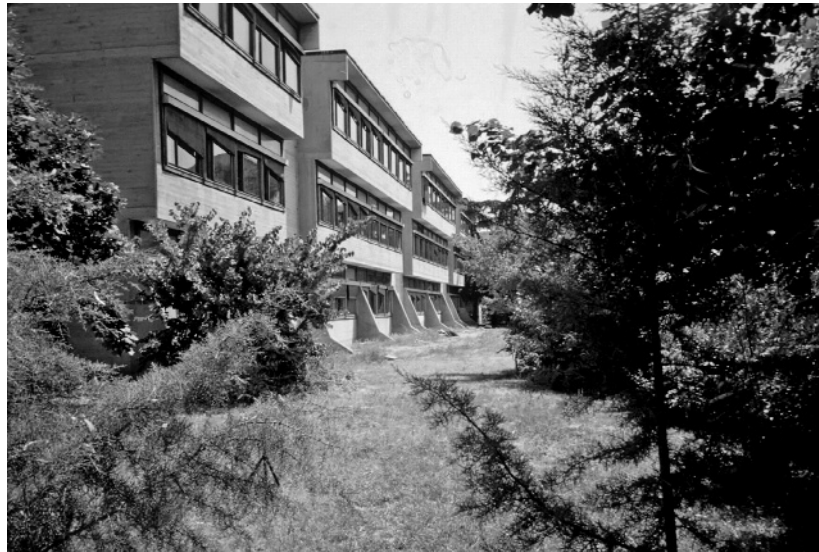
Figure 1.3 The first rubber isolated building: the Pestalozzi elementary school completed in 1969 in Skopje. Courtesy of James M. Kelly, NISEE Online Archive, University of California, Berkeley
