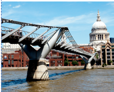
The Millennium Bridge.
