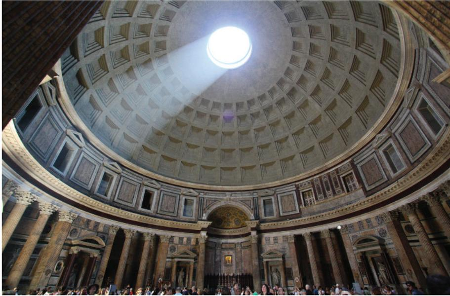
To better manage the weight of the concrete, hard and durable basalt was added to the mix for the foundations, with the mix gradually getting lighter, until pumice rock was used toward the oculus. This way, the base of the dome has the weight and strength to support the rest of the dome, while the upper parts of the dome are thin and light, reducing their load upon the base.
