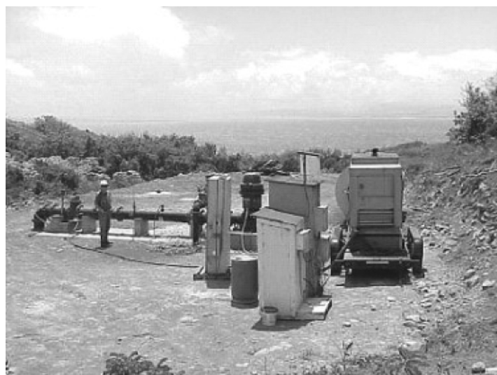
Figure 1.3 A Well Providing about 1.5 MGD (5.68 MLD) of Water to Central Maui, Hawaii (Source: Courtesy of the Department of Water Supply, Maui County, Hawaii, USA)
