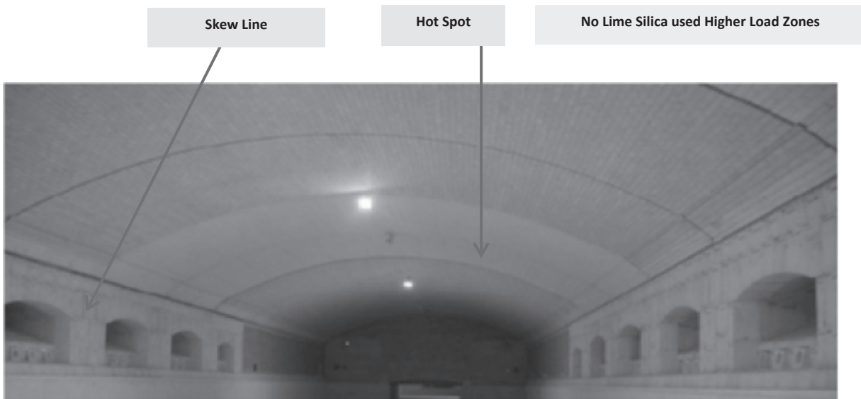
Figure 9. Installation of lime-free-Silica (Stella® GNL) in stressed areas of a regenerative heated float melter
