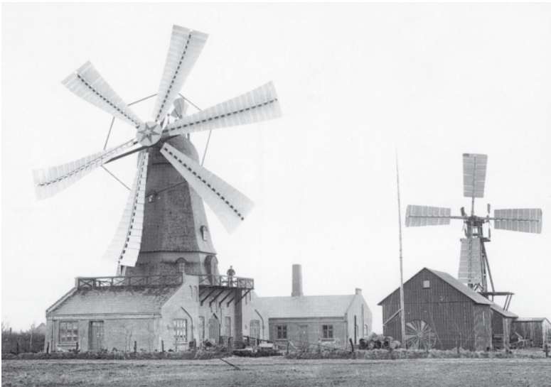
Windmills built by Poul la Cour for generating electricity at Askov, southwestern Denmark. First mill (right) was erected in 1891 and had a diameter of 11.6 m with four flap blades. The second mill (left) was built in 1897 and was 22.8 m in diameter. The picture dates from that year and shows the six-bladed conical wind rotor of Christian Sørensen.
