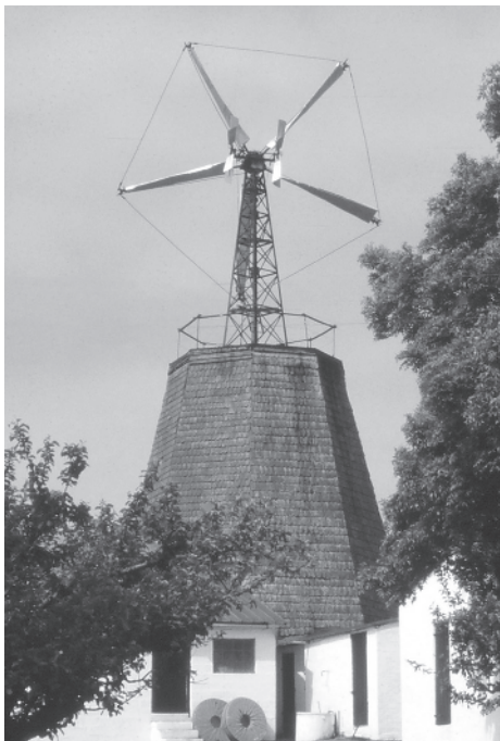
Agricco windmill on the island of Bornholm, Denmark. Five-bladed model with twin fantails erected on the base of an older Dutch-style mill in Olsker. This mill was in service from 1927 until the late 1960s (Christensen 2016). Seen here as it appeared in 1979.
