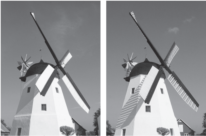
Figure 1.5 Aarsdale Mølle, a smock, Dutch-style windmill on the island of Bornholm, Denmark. (Left) Flap shutters in closed position and blades turning in counterclockwise direction, (Right) flap shutters in open position and blades not turning. Note variation in pitch along length of blades and the fantail on back side of mill. This mill was built in 1877, and the original sail blades were replaced with flap-shutter blades in 1919–1921. The mill still operates today, although not on a regular basis.
