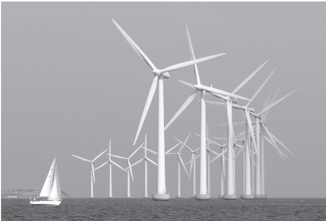
Figure 1.23 Middelgrunden wind farm in the Øresund strait between Denmark and Sweden. A single, curved alignment; commissioned in 2001 with 20 Bonus 2.0 MW turbines. This wind farm is highly visible to the public given its location near Copenhagen, Denmark. Arnoldius/Wikimedia Commons/CC BY-SA 3.0.
