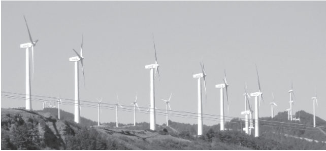
Figure 1.22 EHN turbines harvest wind energy on a prominent ridge near Pamplona, northern Spain. Photo courtesy of J.T. Aber (2012).
