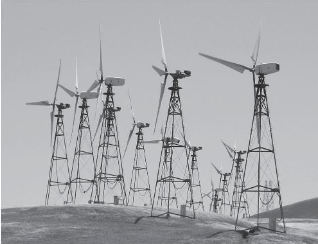
Figure 1.15 U.S. Windpower turbines at Paterson Pass in the Altamont Pass wind-energy complex as seen in 2012. The turbines have three fiberglass blades with variable pitch mounted downwind from the tower. Rotor diameter is 17 m with nominal output of 100 kW (Musgrove 2010).
