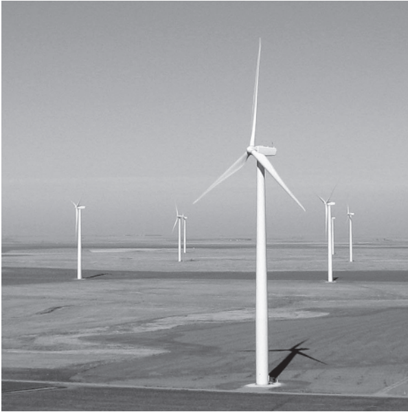
Figure 1.20 Spearville Project, built in 2006, is equipped with GE Wind 1.5 MW turbines amid agricultural fields. These GE Wind turbines were made in the United States; they are descendants of the Tacke turbine made in Germany during the 1990s. Kite aerial photograph with D. Leiker and C. Unruh (2007).
