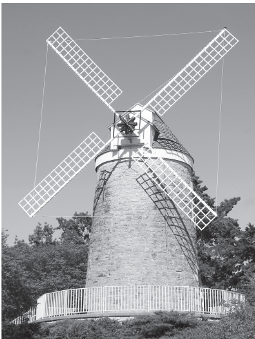
Figure 1.5 Aarsdale Mølle, a smock, Dutch-style windmill on the island of Bornholm, Denmark. (Left) Flap shutters in closed position and blades turning in counterclockwise direction, (Right) flap shutters in open position and blades not turning. Note variation in pitch along length of blades and the fantail on back side of mill. This mill was built in 1877, and the original sail blades were replaced with flap-shutter blades in 1919–1921. The mill still operates today, although not on a regular basis.
