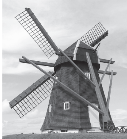
Figure 1.3 Klostermøllen near Vestervig in northwestern Jutland, Denmark. A typical Dutch-style windmill; it was built in 1860 and continued in service until 1960. The mill was restored to its original state in the late 1980s. Further restorations were necessary after storm and lightning damages.
