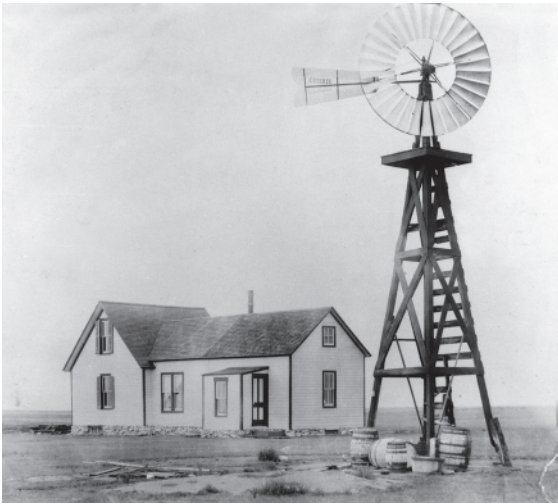
Historic farmstead of D.R. Beckstrom, who moved to Greeley County in westernmost Kansas in 1892 (C. Shepherd, pers. com. 2023). The Currie windmill has a large wheel with 30 blades. Notice the wooden water barrels at the bottom. The mill presumably dates from the 1890s, as it appears to show Manhattan as the manufacturing city. Undated image obtained from the Horace Greeley Museum in Tribune.
