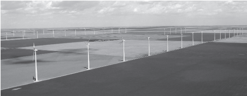
Figure 1.19 Gray County Wind Farm, built in 2001, was the first large array of turbines in Kansas. It has 170 Vestas V47 turbines with a combined capacity of 112 MW. These turbines are relatively small and closely spaced compared with newer models. Kite aerial photograph (2006).
