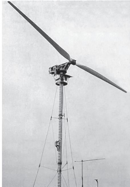
Figure 1.11 Allgaier–Hütter StGW-34 model, two-bladed, 100 kW wind turbine located at Stötten, ~80 km east of Stuttgart, Germany (1958). With a rotor diameter of 34 m, it was the first turbine with fiberglass blades. Courtesy of H.H. Dörner.
