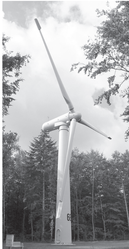
Figure 1.17 Vindeby turbine preserved and displayed in the Danish Energy Museum. Blades are 17 m long, the tower originally stood 33 m tall, and generating capacity was 450 kW. Note the brake flaps in the blade tips. From the world's first offshore wind farm erected in 1991 and taken offline in 2017.
