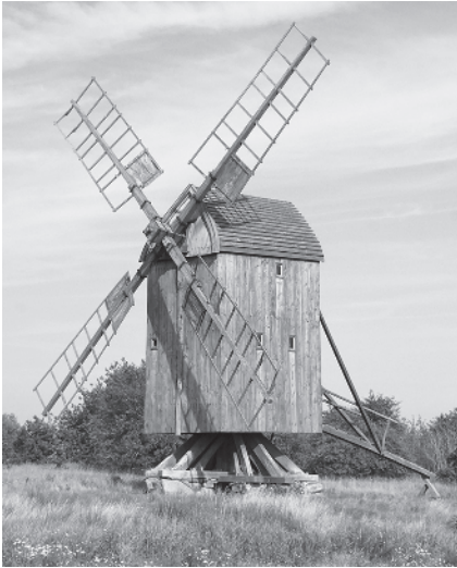
Figure 1.2 Egeby Stubmølle (post mill) was built in 1787. The mill is rotated manually with the long tail pole (to right). It is no longer in service, but has been restored and functional since 1999. Island of Bornholm, Denmark.
