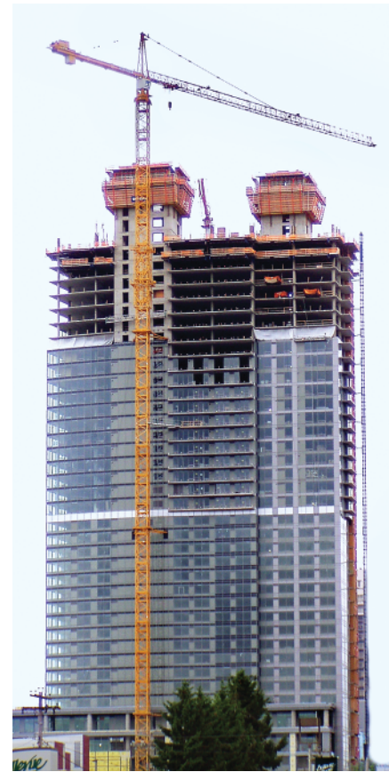
FIGURE 1.12 In this photo, the construction sequence of a tall building is readily apparent: A pair of concrete core structures leads the construction, followed by concrete columns and floor plates and, finally, the enclosing curtain wall. (Photo by Joseph Iano.)
