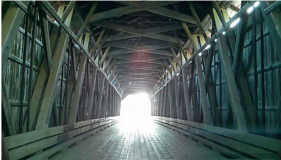
Figure 1.18 A Howe truss-type covered bridge in Quebec, Canada.
