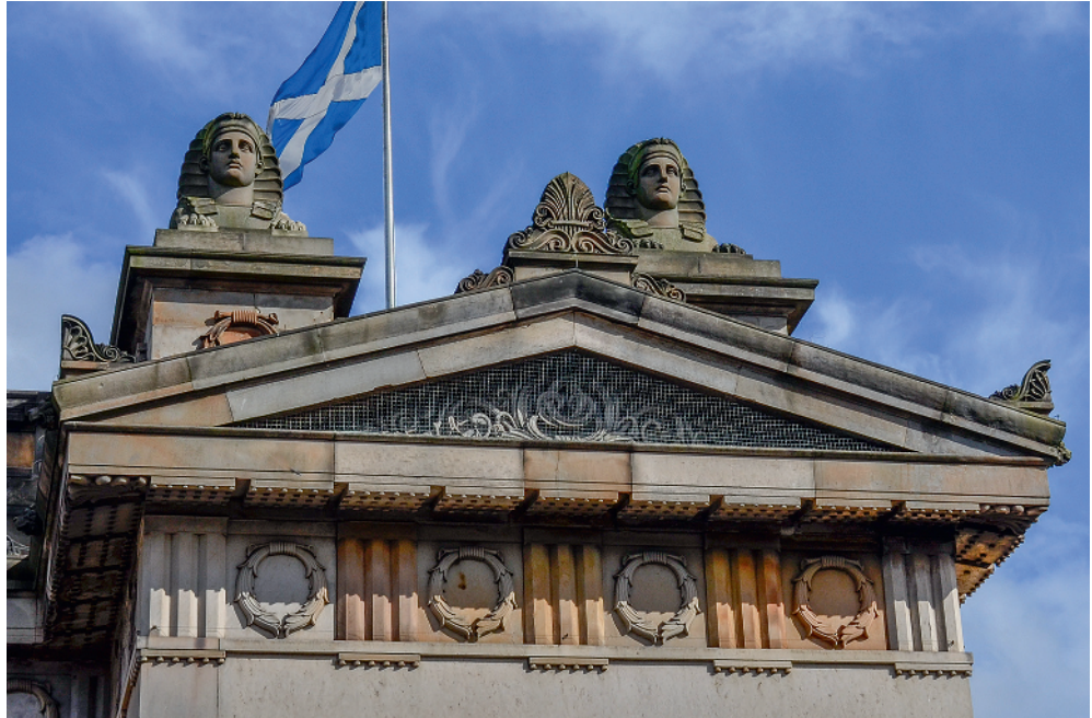
Figure 1.5 Triglyphs (on the frieze) and dentils (above it) decorate this neoclassical façade in Edinburgh, Scotland.
