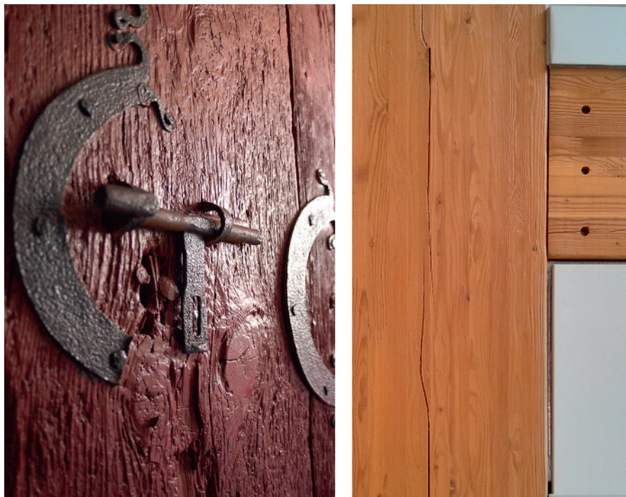
Figure 1.1 Hundreds of years lie between these two wood surfaces. One (on the left) is a medieval solid wood door, and the other (on the right) is a contemporary glulam structure.
