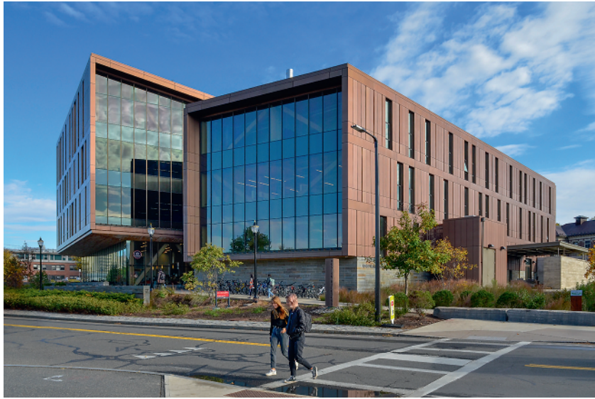
Figure 1.25 The John W. Olver Design Building at the University of Massachusetts in Amherst, MA. This 87,500-ft 2 mass timber building features a glulam frame, CLT floors, roofs, and shear walls, as well as a wood-concrete composite flooring system. Interior views of this project will be visible in many locations in this book.
