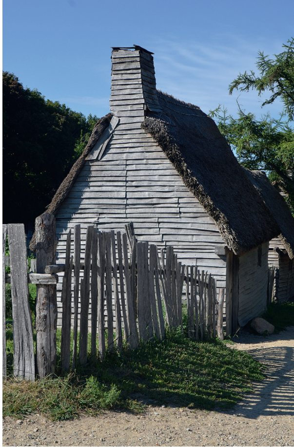
Figure 1.10 An early version of clapboard siding is being demonstrated in this reconstructed house in Plymouth, Massachusetts.
