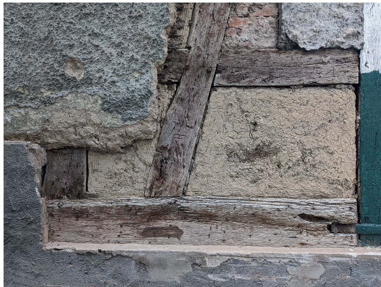
Figure 1.9 Wall section of a half-timbered house under renovation. Between the wood frame is a wattle and daub wall infill, and on top of it is a plaster render (visible at the top left).
