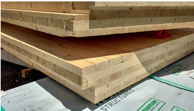
Figure 1.23 Cross-laminated timber panels at a construction site.
