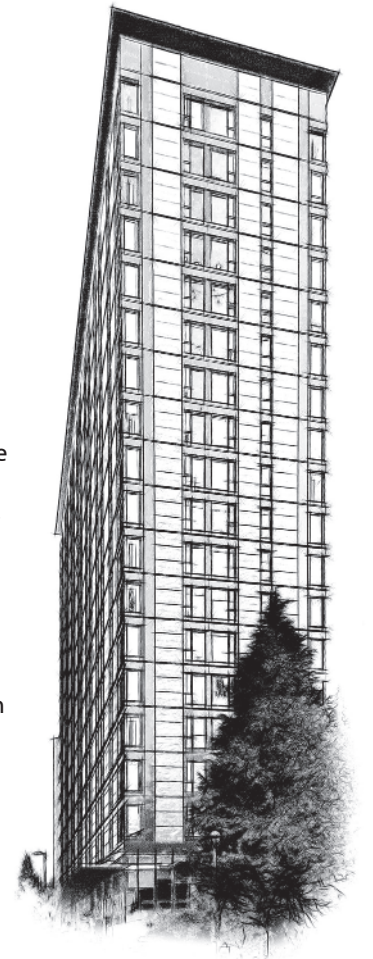
Figure 1.25 The John W. Olver Design Building at the University of Massachusetts in Amherst, MA. This 87,500-ft 2 mass timber building features a glulam frame, CLT floors, roofs, and shear walls, as well as a wood-concrete composite flooring system. Interior views of this project will be visible in many locations in this book.
