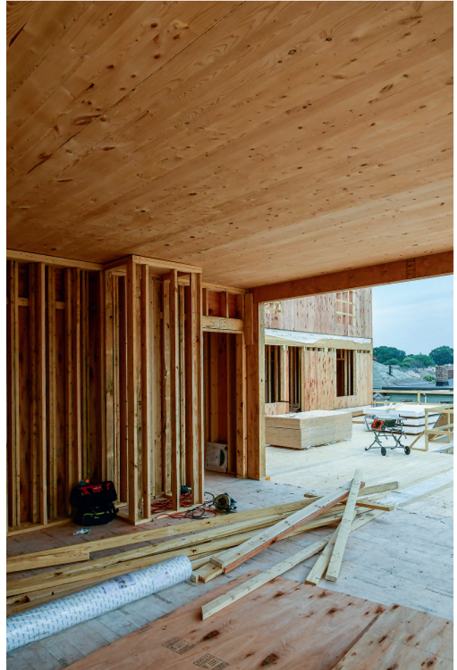
Figure 1.29 A project in Somerville, MA, is using CLT made from a non-traditional species: Eastern Hemlock.
