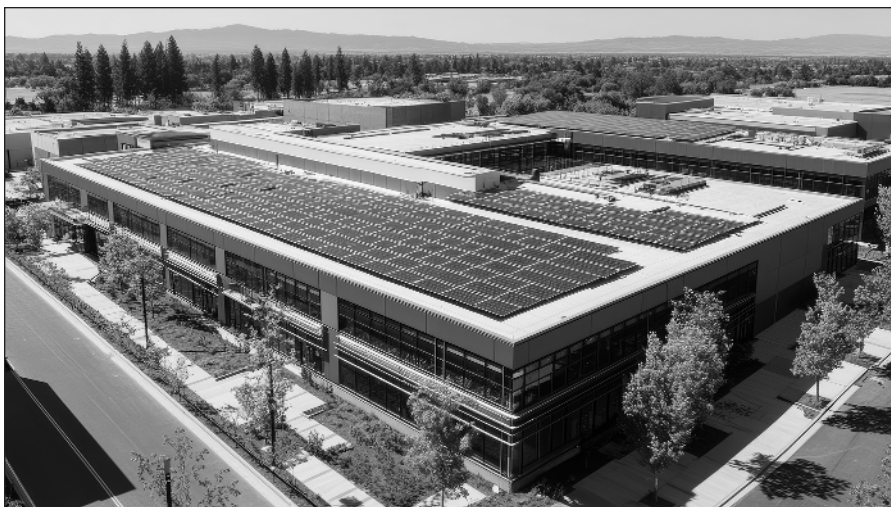
FIGURE 1-3: Solar panels sprawling across the rooftop of a business.
