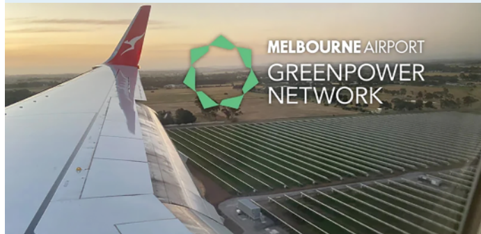
FIGURE 7 Melbourne Airport is developing a solar panel network designed to generate enough energy to power all of its terminals.
