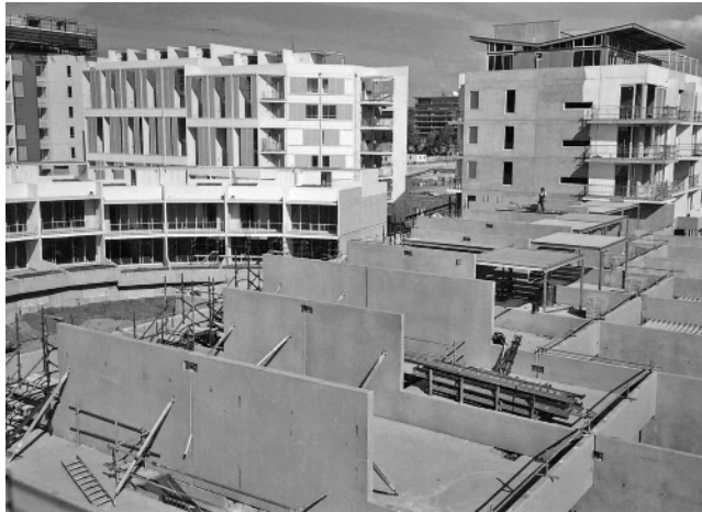
Figure 1.18 Wall frames used in apartment buildings and retail units near Sydney.
