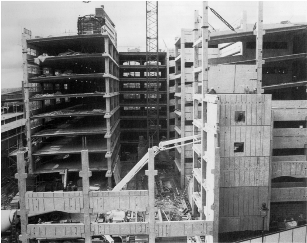
Figure 1.38 Construction sequence block by block (courtesy of Blatcon Ltd).
