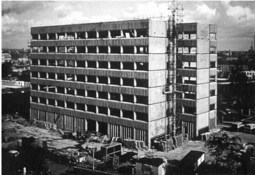
Figure 1.4 Precast construction of the 1960s using the National Building Frame, The building is Highbury College, now part of the University of Portsmouth (courtesy of Costain Building Products).
