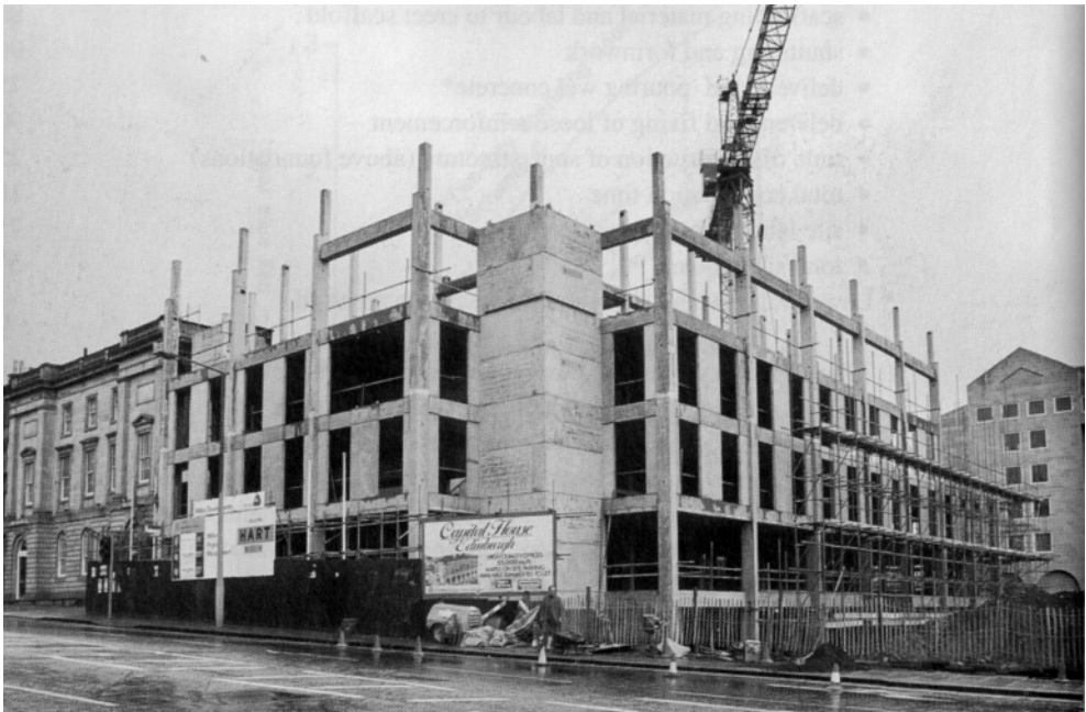
Figure 1.37 Construction sequence floor by floor (courtesy of Trent Concrete Ltd).
