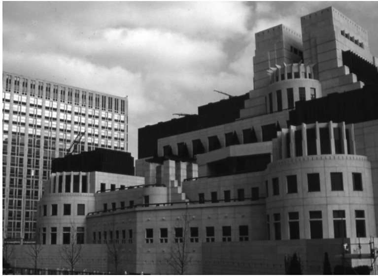
Figure 1.12 Examples of past and present use of precast concrete, Vauxhall Bridge, London.
