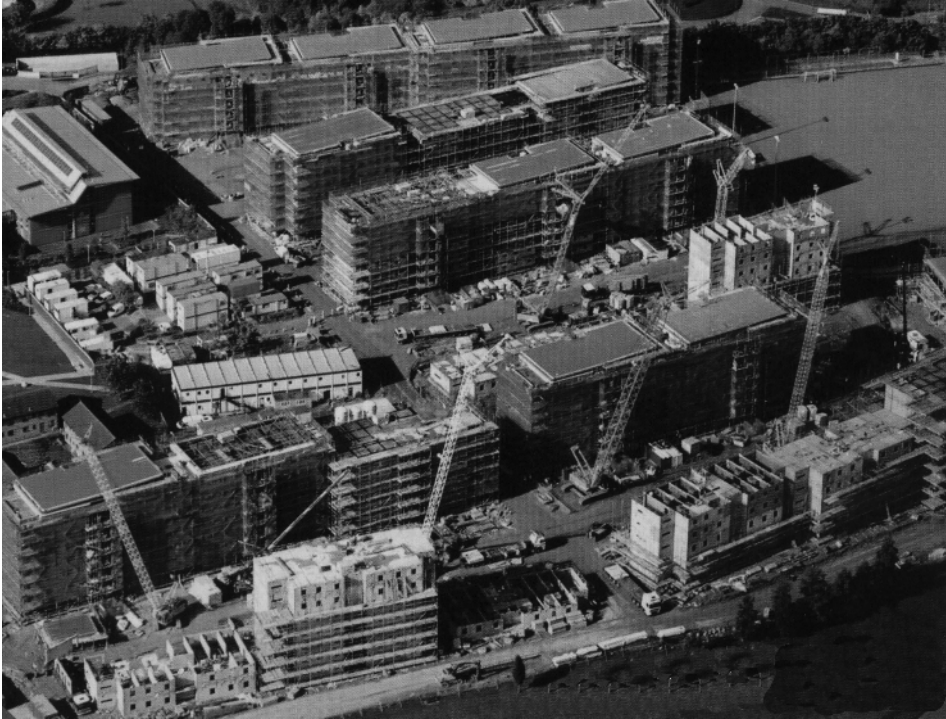
Figure 1.11 Student accommodation buildings at the University of West of England, Bristol. Precasted by Buchan, UK.
