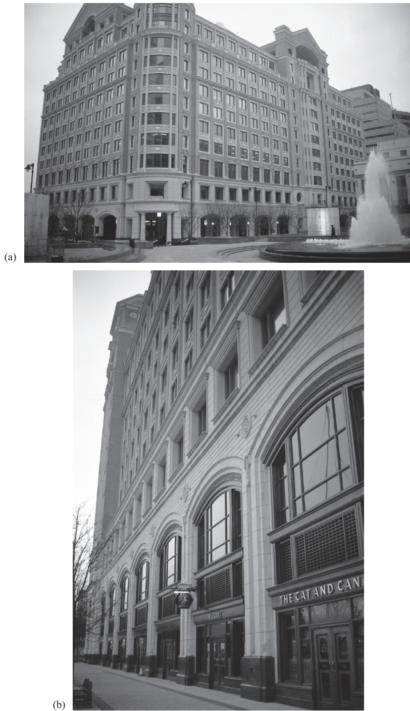
Figure 1.6 An early example of quality architecturally detailed precast concrete imported from Belgium. (a) Overall impression. (b) Architectural detail. (Courtesy of A. Van Acker, TU Ghent.)
