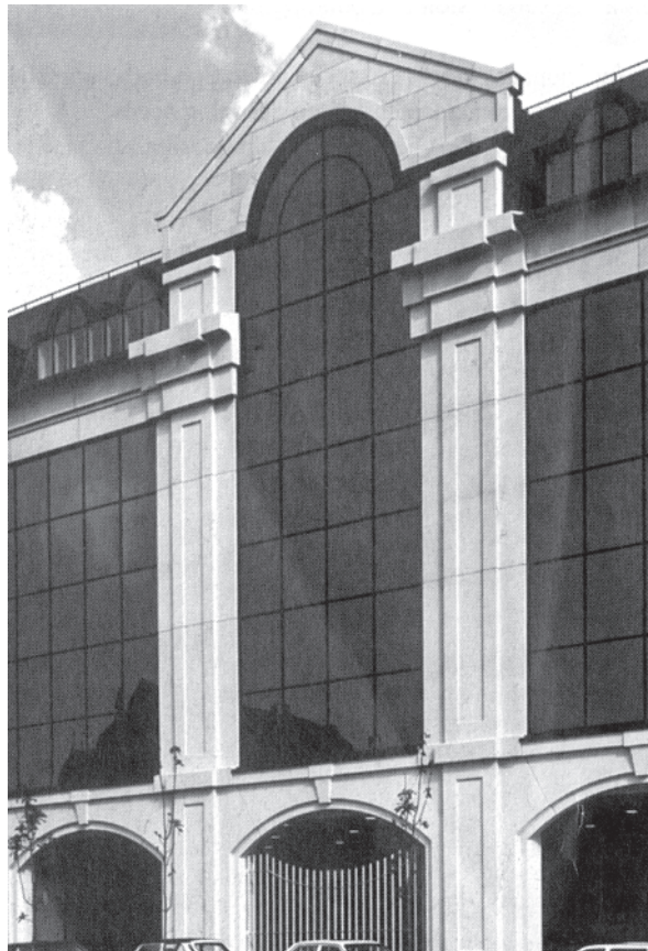
Figure 1.13 Principle of the twin facade system: (a) diagrammatic representation and (b) offices, Brussels.
