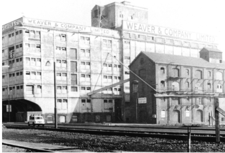
Figure 1.1 Weaver's Mill, Swansea – the first precast concrete skeletal frame in the United Kingdom, constructed in 1897–98 (courtesy of Swansea City Archives).
