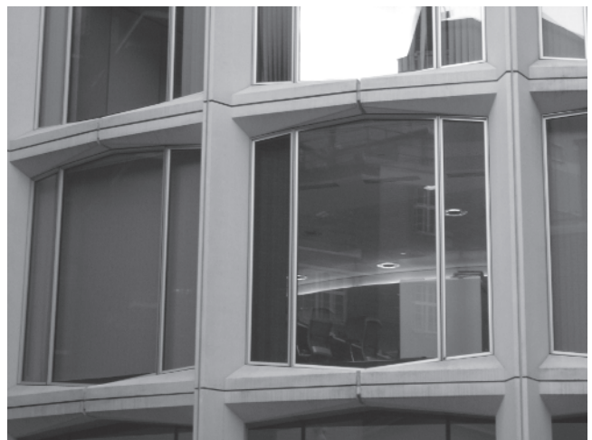
Figure 1.10 Asticus Building, London, 2010. Precast cruciforms form (a) the exterior structure, and (b) architectural finish.
