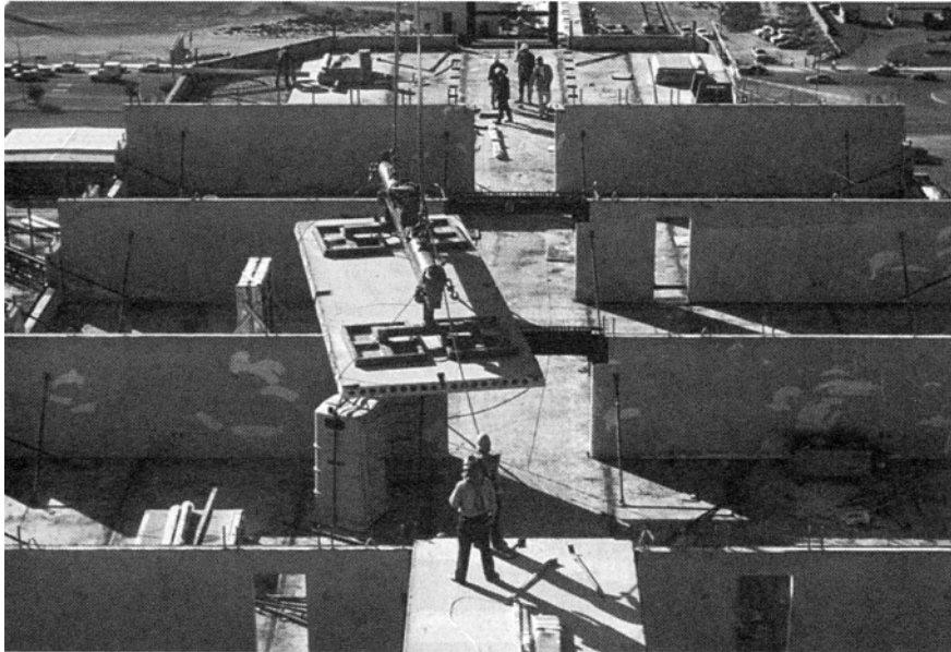
Figure 1.7 MGM Hotel and Casino at Las Vegas, US constructed in 1992 (courtesy of A. T. Curd).
