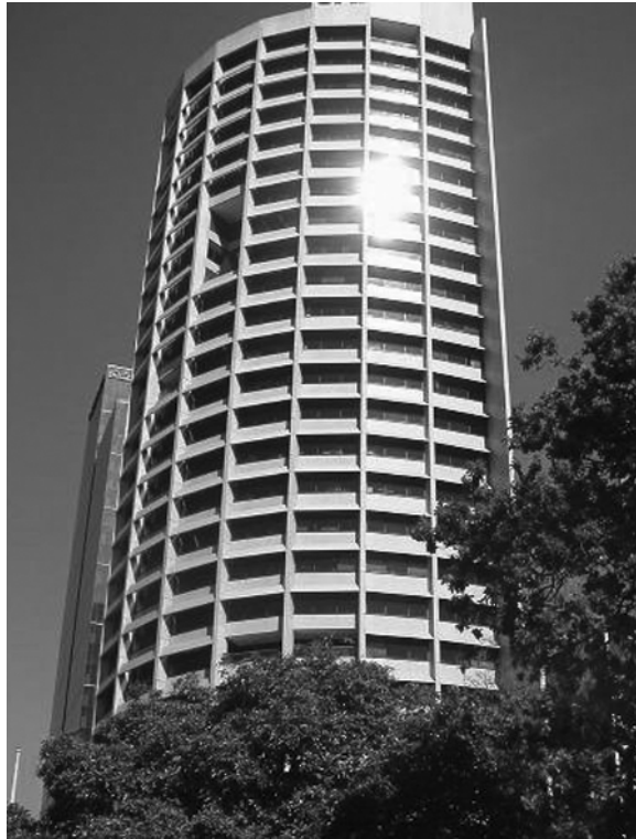
Figure 1.9 Granite aggregates in spandrel beams and columns, polished to reflect the Australian sunshine at No. 1 Spring Street, Melbourne, 1990.
