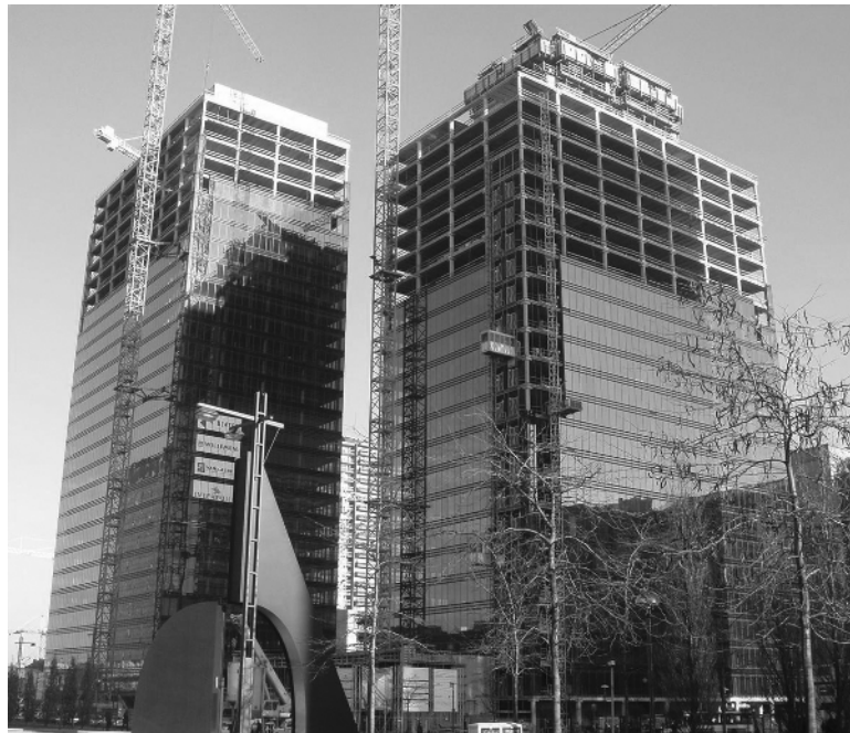
Figure 1.8 36-storey precast skeletal tower buildings in Brussels (courtesy of Ergon, Belgium).
