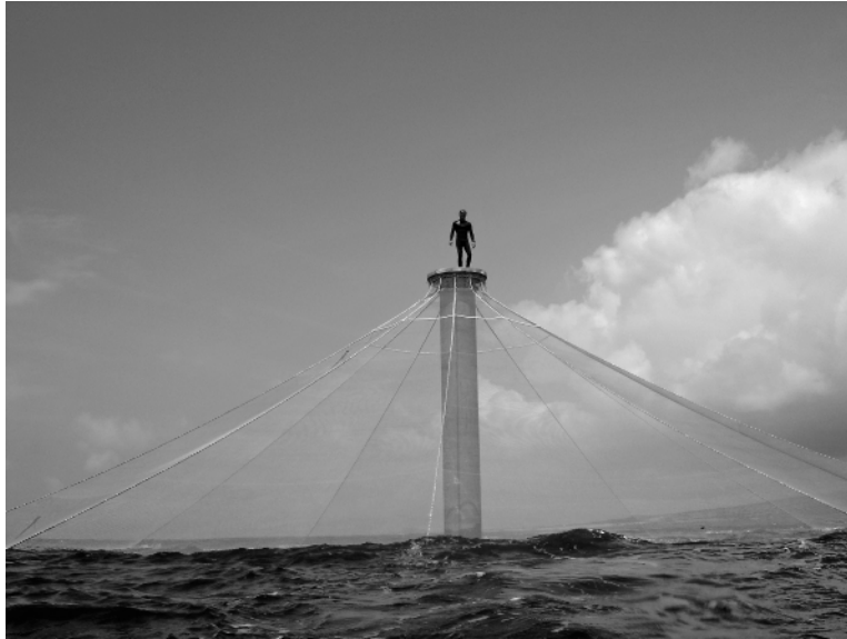
Fig. 1.6 Sea Station 3000 is a fully submersible 3000m 3 seacage (24m diam × 16.5m tall). In operation the seacage is submerged to below 10m depth, ca. 800m off the Kona Coast of the Big Island of Hawaii. It is stocked with up to 70000 Seriola rivoliana (see cover photograph). The Offshore Site Manager is standing on the spar of the semi-submerged structure. (Photograph from Kona Blue Water Farms, Inc. Kona Kampachi®.)
