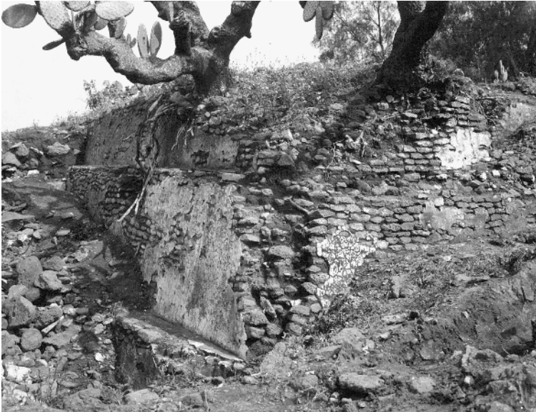
Figure 1.9 A small temple platform at the site TA-8 in the Teotihuacan Valley. This structure was built of small stones and covered with white lime plaster. It was discovered by a regional survey project directed by William T. Sanders (Evans and Sanders 2000:115)
