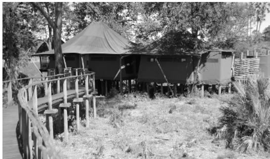
Figure 1-19. Ecotourism camp in the Okavango Delta of Botswana. The tent structures are elevated on wooden posts to minimize surface impact, and the interior accommodations are quite comfortable. Photo courtesy of M. Storm.
