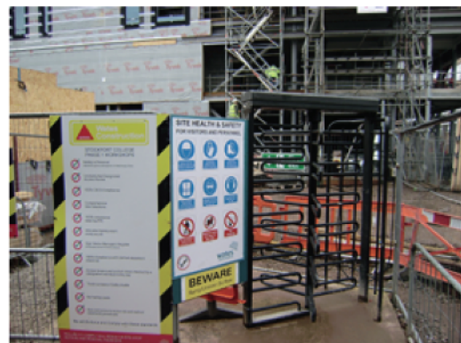
Gate entry to site
