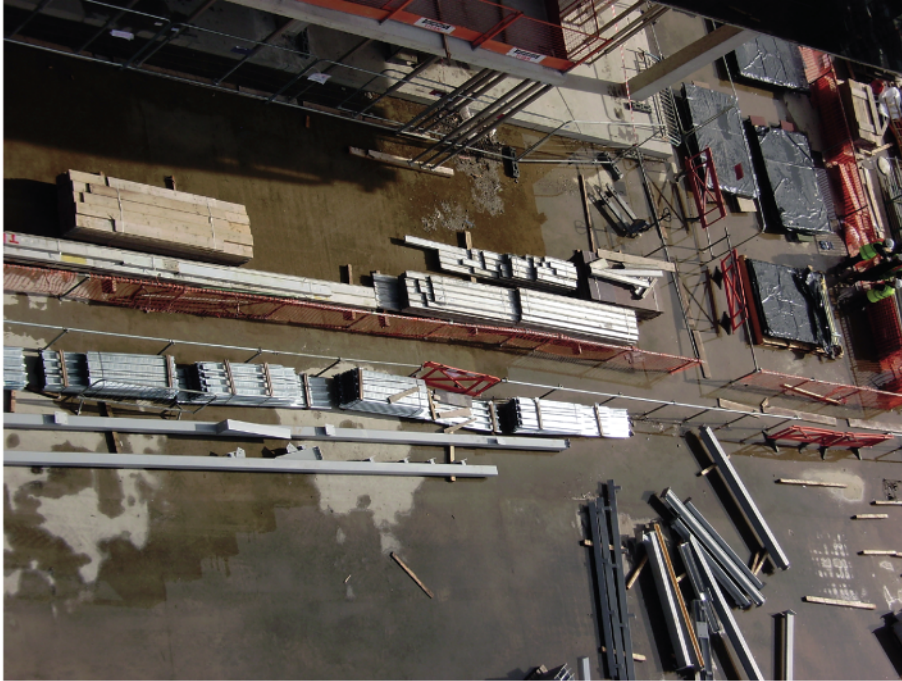
Site storage area for storey height granite external cladding panels
