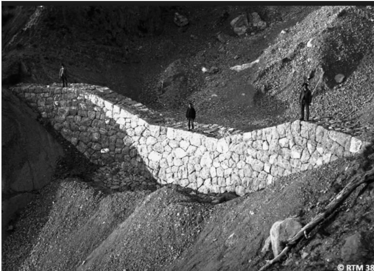
Figure 1.12. Dam no. 1 on the Pravert torrent, built in 1894 in Tréminis (Dévoluy, Southern Alps) (source: RTM 38)
