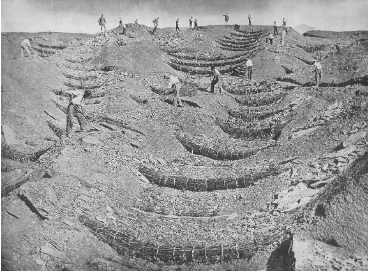
Figure 1.11. Stabilization of a basin head with a substrate composed of marl and limestone through the riverbanks' shaping and the fixation of "living fascinings" (bundles of sticks meant to take root), the area of the Curusquet in Basses-Alpes (source: Archives RTM)
