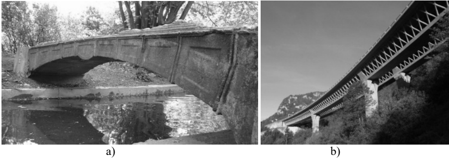
Figure 1.1. a) The first cast cement bridge (Louis Vicat, Grenoble, 1853); b) the Glacières Viaduct (France, 1988), truss structure in prestressed concrete (source: P. Paultre and J. Mazars). For a color version of this figure, see www.iste.co.uk/mazars/damage.zip
