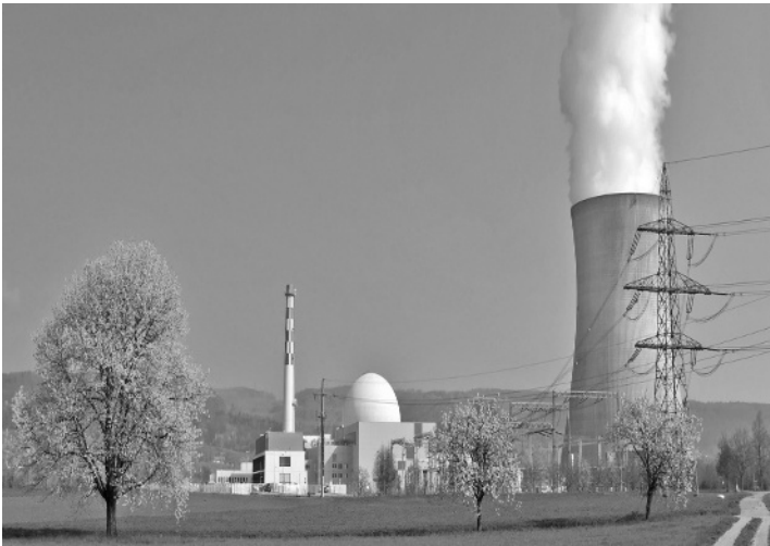
Figure 1.6. Nuclear power plant
