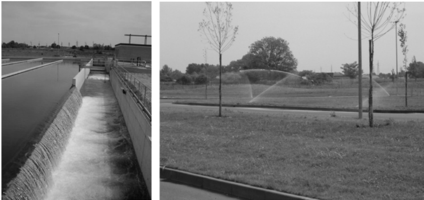
Figure 1.5. On-site spraying with reused water (Nosedo)
