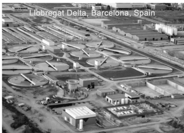
Figure 1.10. Barcelona plant with tertiary treatment
