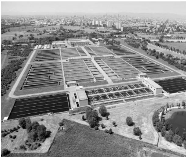
Figure 1.4. Nosedo wastewater treatment plant including tertiary treatment
