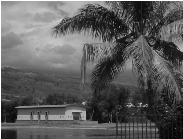
Figure 1.8. Tertiary treatment plant (Reunion Island, France)
