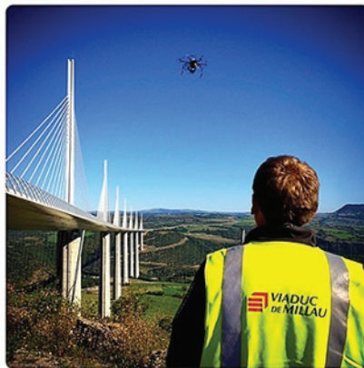
Figure 1.7. Diagnostic of Millau viaduct performed by drone (source: Eiffage CEVM/Foster + Partners/DIADES)
