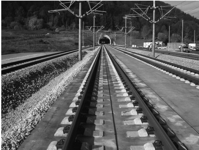
Fig. 1.9 Rheda 2000 system (source: Institute of Road, Railway & Airfield Construction, Munich TU)
