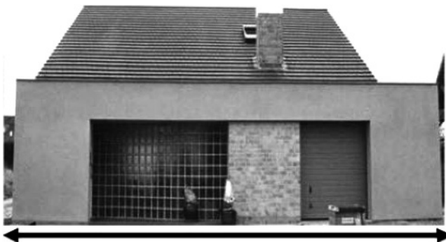
Fig. 1.38 The arrow shows a part of the free perimeter
