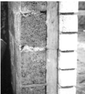
Fig. 1.4 Filled cavity wall
