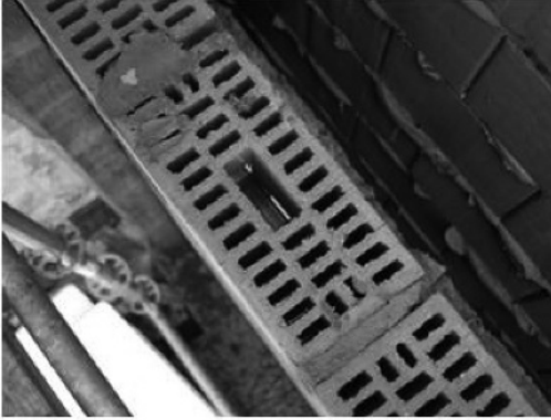
Fig. 1.32 Masonry, clearly not a layer where the heat flux develops one-dimensionally
