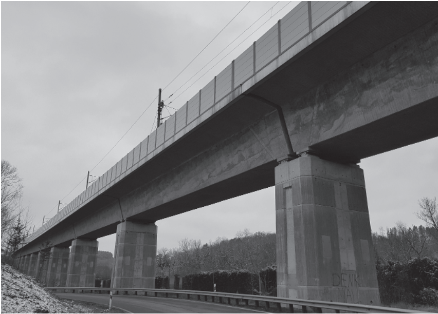
Figure 1.2 Railway concrete bridge with uniform single span girders and compact columns.
