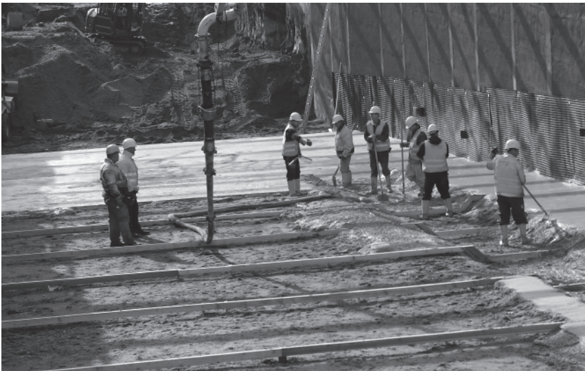
Figure 1.9 Workers manually distributing and planning a concrete subbase.
