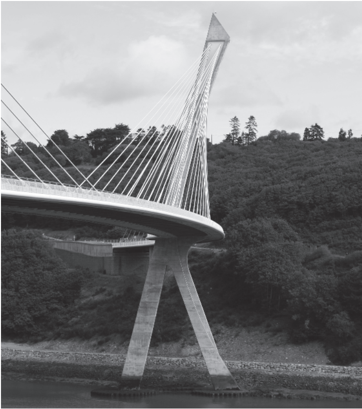
Figure 1.1 Concrete shaped to the flow of forces: pylon of the Pont de Terenz (France). Picture: Thomas Putke-Hohmann.
