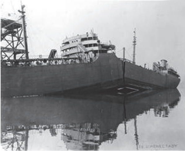
Figure 1.2 The Schenectady after it broke into two on January 16, 1943, in dock in Portland, Oregon. The ship had just been finished and was being outfitted. The failure was sudden and unexpected.
