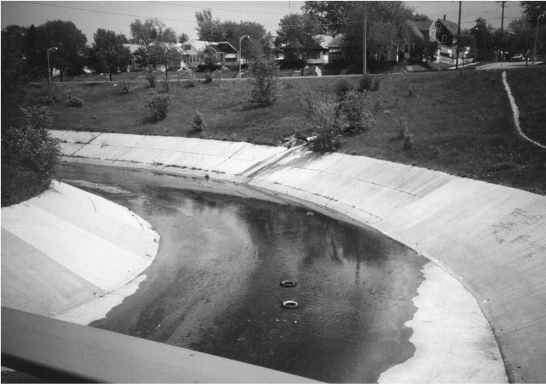
Figure 1.5. Lincoln Creek in Milwaukee lined with concrete, resulting in a loss of habitat. Early in the 2000s, the lining was removed and creek habitat was restored.
