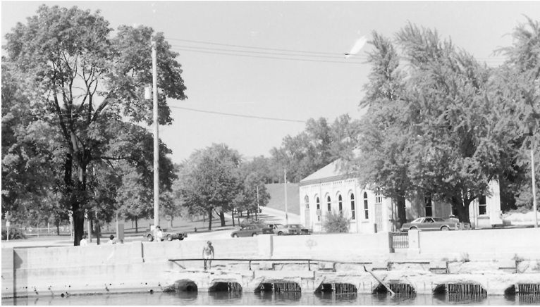
Figure 1.2. Intake to the flushing tunnel and pumping station are the national civil engineering landmark in Milwaukee, Wisconsin. The pumping station is more than 100 years old. A large quantity of flow is pumped into the Milwaukee River upstream from the harbor during periods of dissolved oxygen deficiency.
