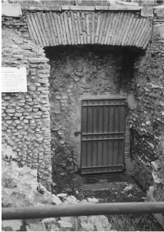
Figure 1.1. Stormwater inlet into the ancient Roman sewer cloaca maxima at the Forum Romanum in Rome.
