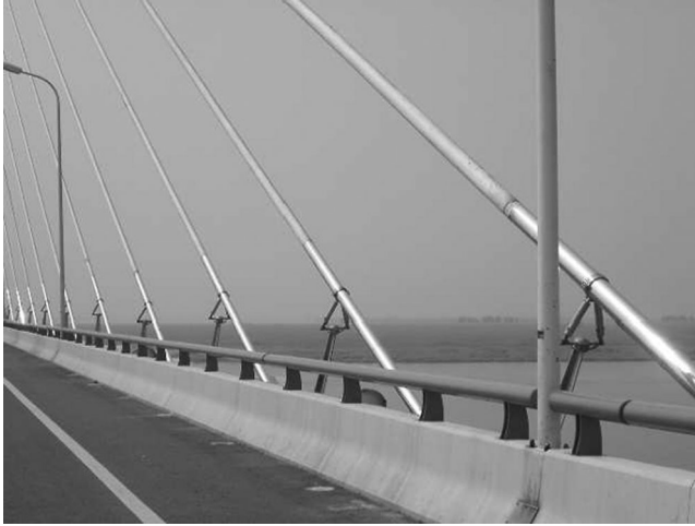
Figure 1.19 Damper configuration (Spencer, 2002)
