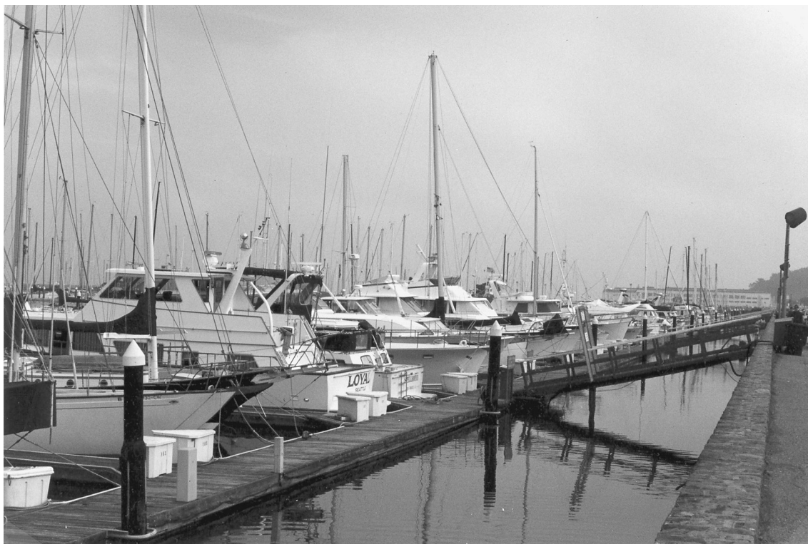
Figure 1.21 Articulated access ramp to a floating dock.
