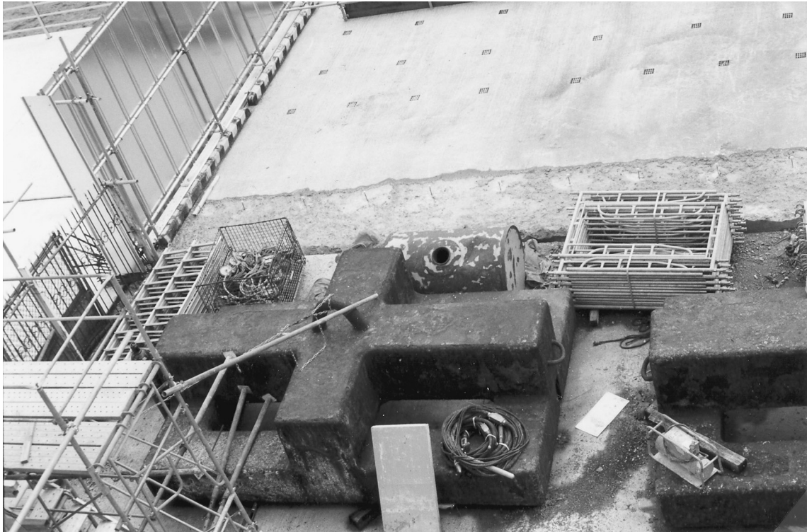
Figure 1.22 Raw iron gravity anchor used for anchoring of floating docks.
