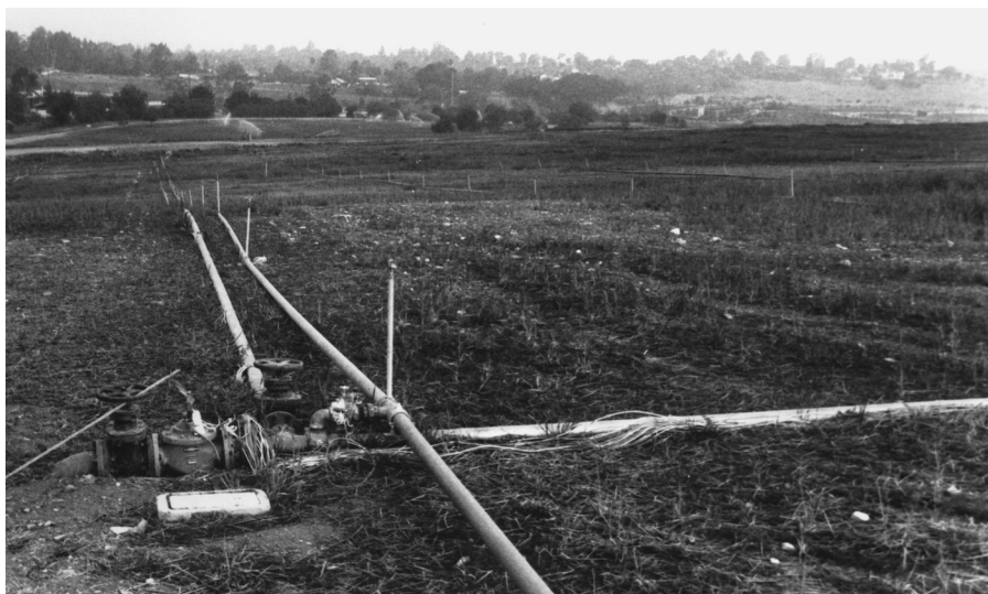
Figure 5-38 Completed landfill with irrigation system.
