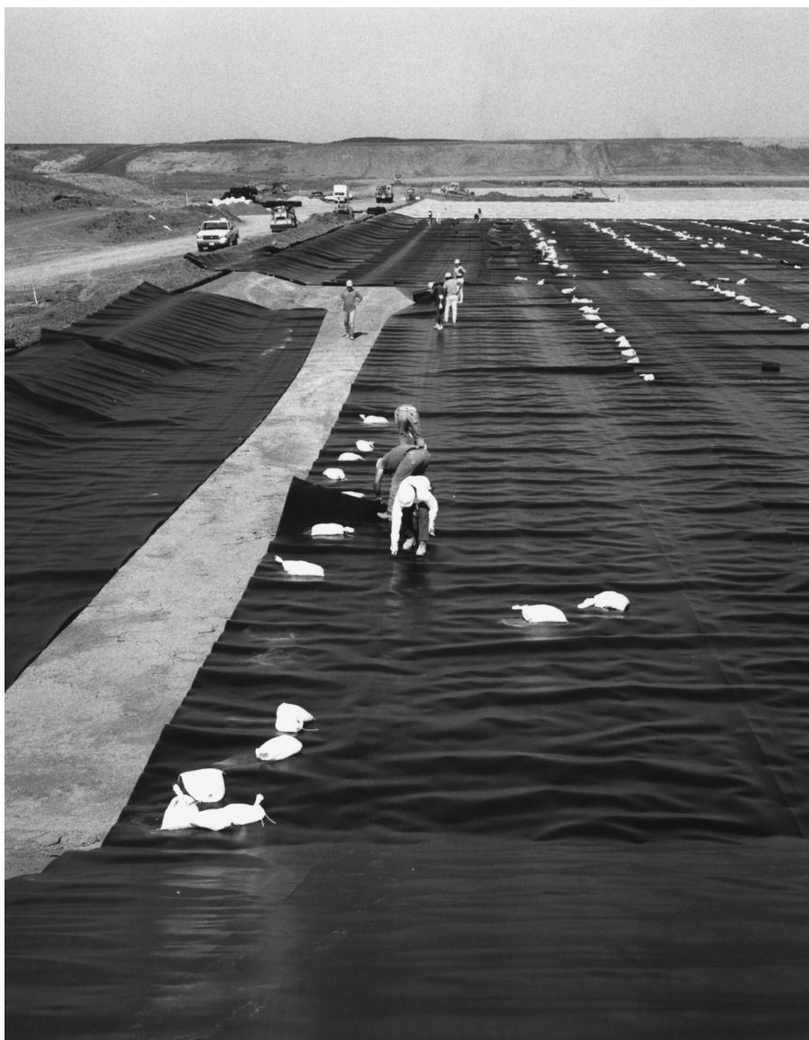
Figure 5-28 Placement of geomembrane liner in area-type landfill.
