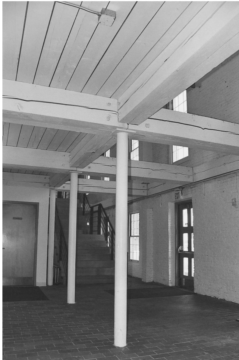
Figure 1-18 Adaptive reuse of mill building, Lowell, Massachusetts. The steel columns, heavy wood beams, brick floor and walls, and wood plank ceiling of this building can be incorporated into designs for a variety of new uses.
