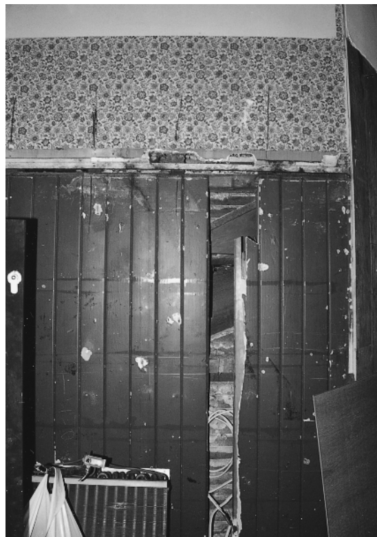
Figure 1-17 The actual composition of a wall in an existing building is sometimes unknown until demolition begins, as is the case here. Discrete removal of outer layers can provide a glimpse of what is behind.
