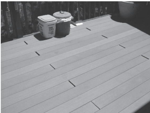
Figure 1.28 Shrinkage of WPC boards.
