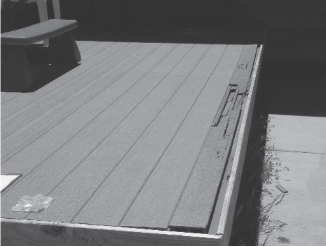
Figure 1.43 An advanced step of crumbling of Mahogany tongue-and-groove composite deck board (Arizona).
