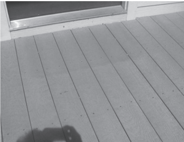
Figure 1.1 Fading of a composite deck. The “Welcome” mat is just removed.
