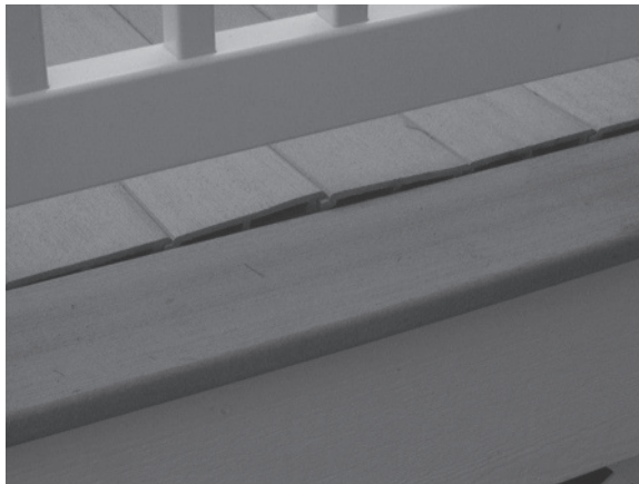
Figure 1.31 A typical appearance of a composite deck in case of buckling or thermal expansion of WPC boards.
